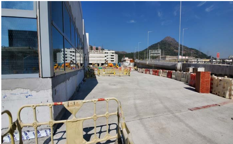
Photo 2 - Construction works at Maintenance Depot
