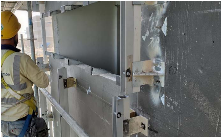
Photo 3 - Construction works at Fire Services Department Building
