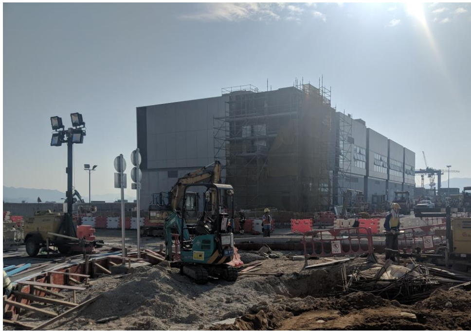
Photo 2 - Site condition at Administration Building
