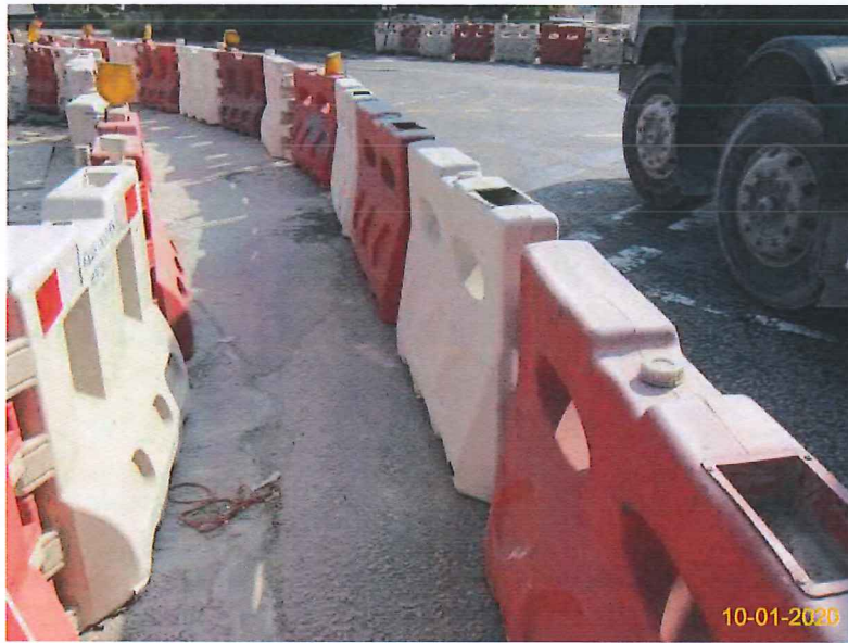
Item 6. Temporary traffic management lighting.
