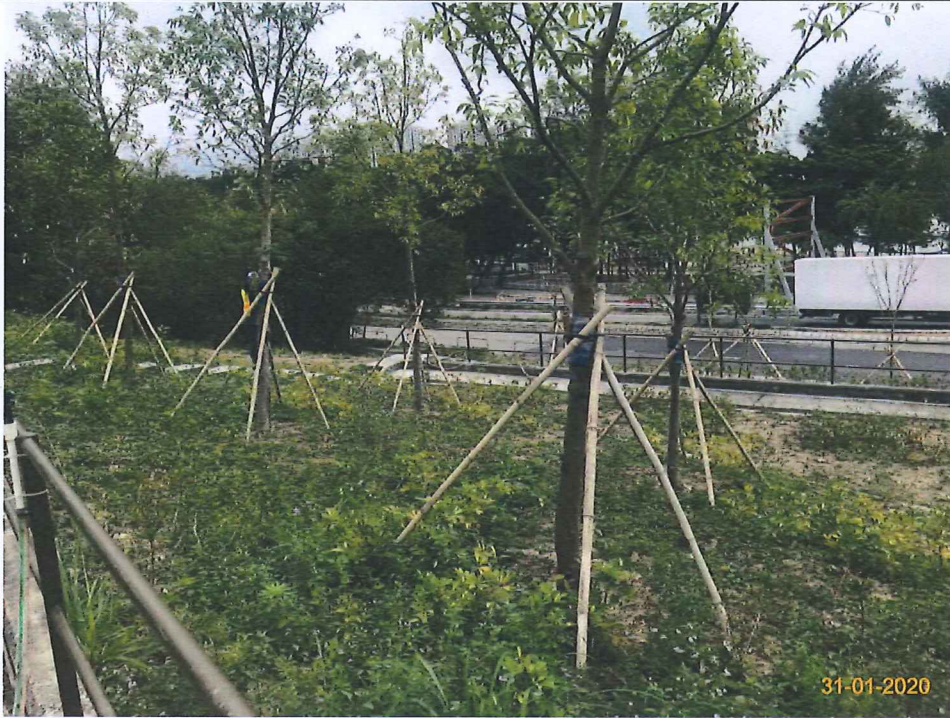
Item 3. Landscape works was commenced.
