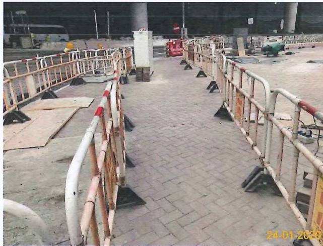
Item 6. Temporary traffic management lighting.
