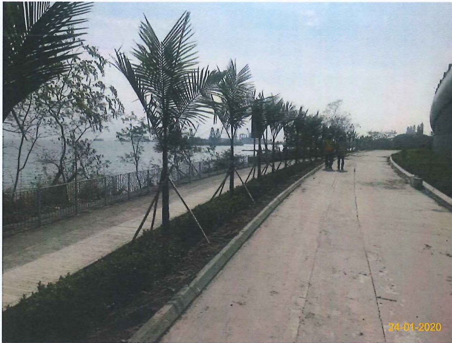
Item 3. Landscape works was commenced.
