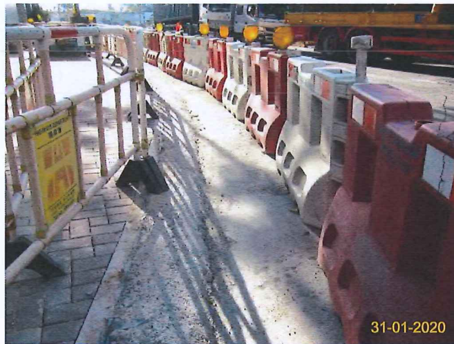
Item 6. Temporary traffic management lighting.
