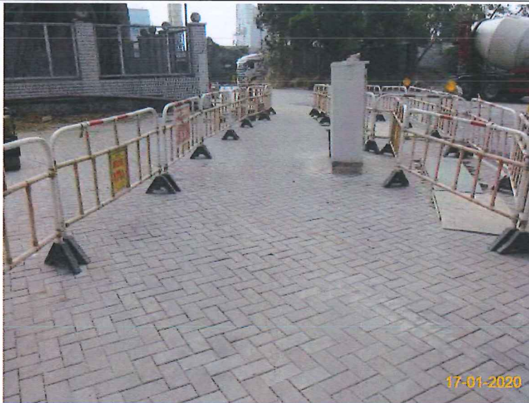
Item 6. Temporary traffic management lighting.
