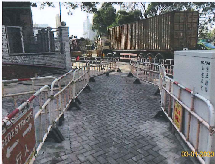
Item 6. Temporary traffic management lighting.
