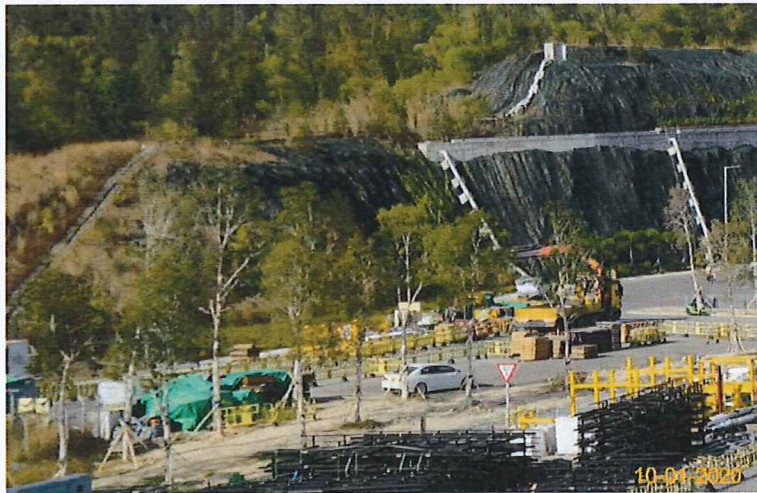
Item 2. Tree Transplanting works conducted on 22-May-17.
