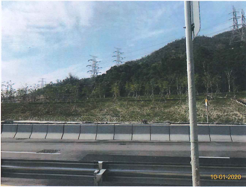
Item 3. Landscape works was commenced.
