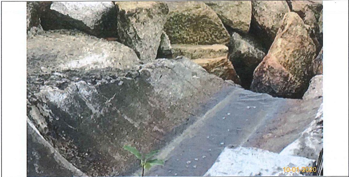
Item 7. Ensure no run-off into water body.(Outfall 1)
