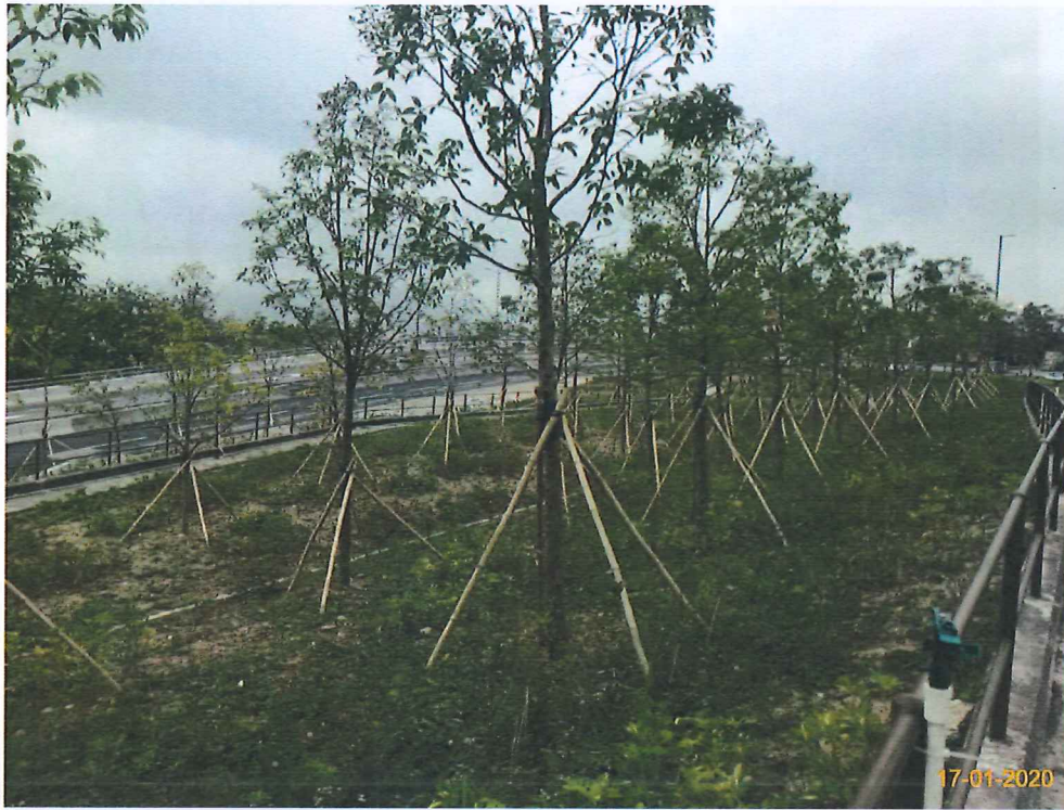
Item 3. Landscape works was commenced.
