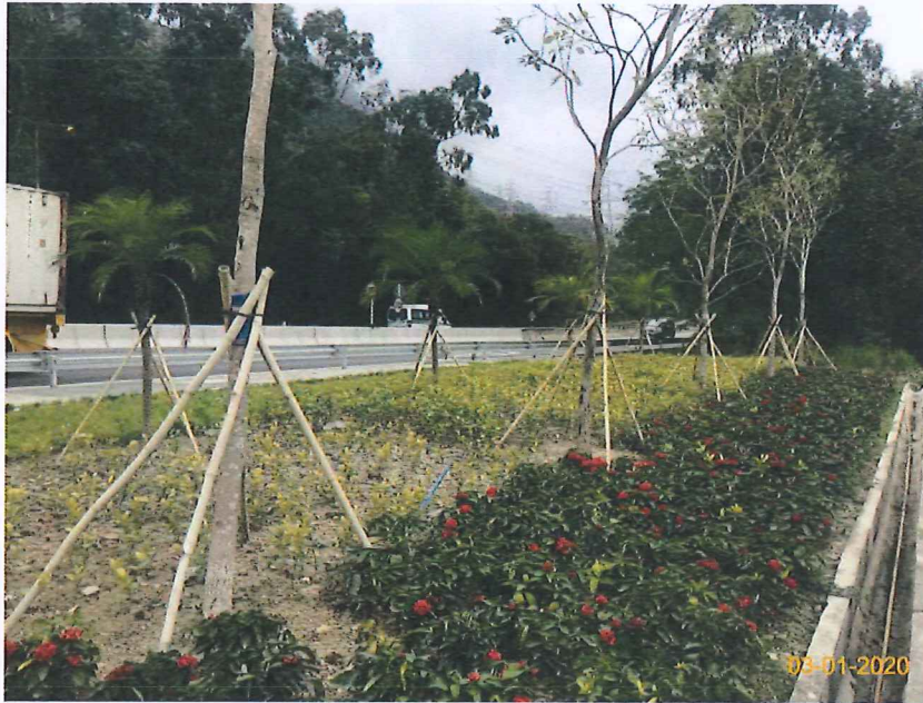
Item 3. Landscape works was commenced.
