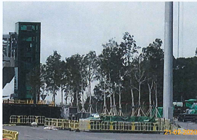
Item 2. Tree Transplanting works conducted on 22-May-17.
