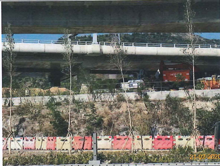
Item 3. Landscape works was commenced.
