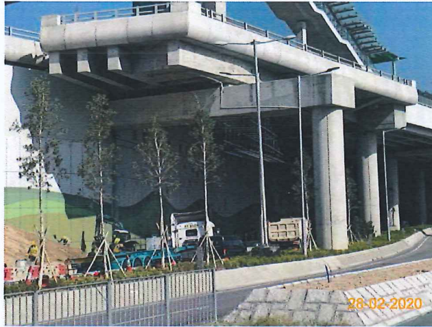
Item 3. Landscape works was commenced.
