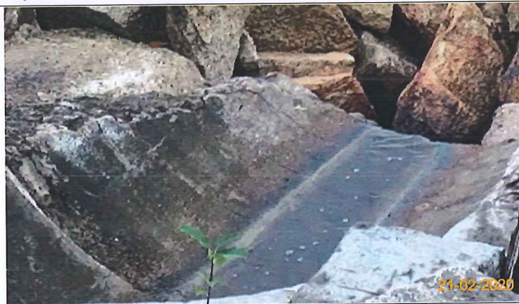
Item 7. Ensure no run-off into water body.(Outfall 1)
