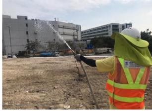
**Photo 8** During the joint site inspection on 17 March 2020 water spraying had been provided for the exposed area to reduce dust impact.
