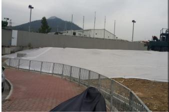
**Photo 9** During the joint site inspection on 17 March 2020 exposed slope had been covered with tarpaulin to reduce dust impact.
