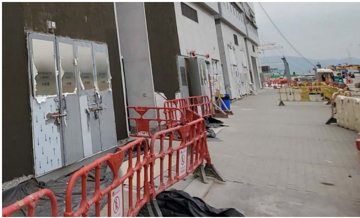
Photo 1 - Construction works at Administration Building
