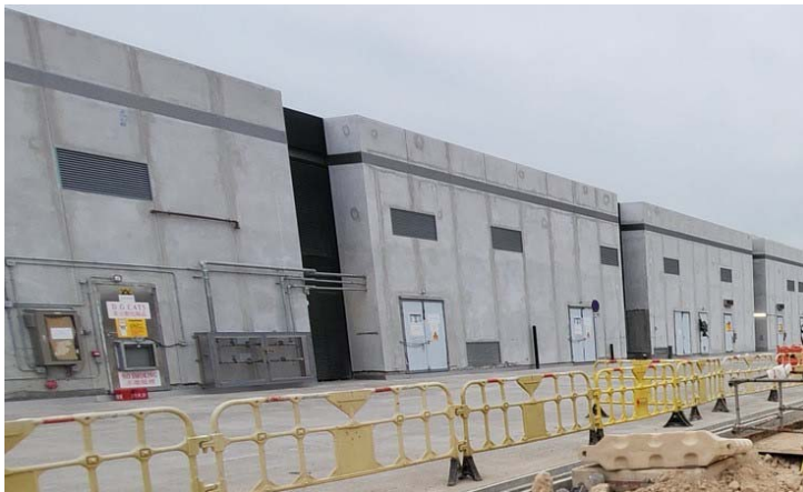
Photo 2 - Construction works at Maintenance Depot
