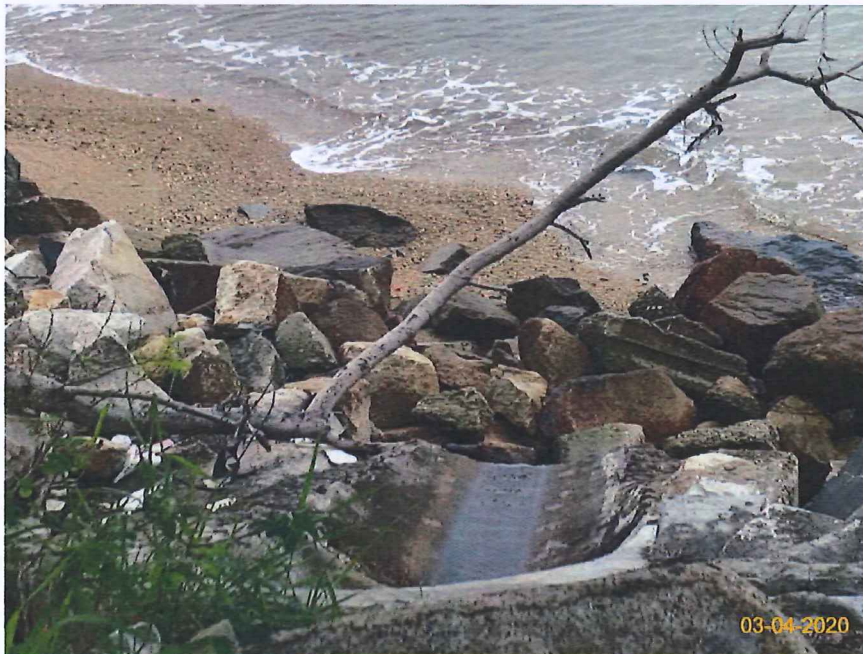
Item 7. Ensure no run-off into water body.(Outfall 1)
