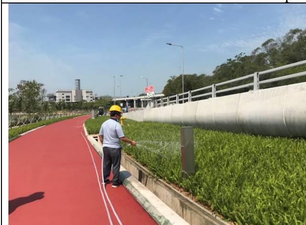
Photo 11 Planting works at Lung Mun Road
