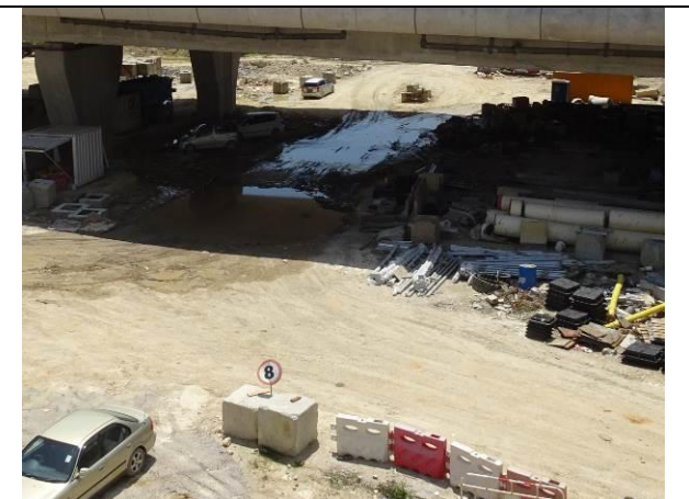
Photo 6 All vehicles using the haul road had enhanced to control the speed below 8km/hr to reduce dust emission.
