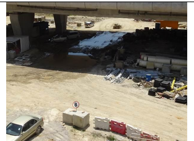
Photo 6 All vehicles using the haul road had enhanced to control the speed below 8km/hr to reduce dust emission.
