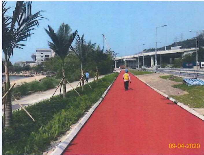
Item 3. Landscape works was commenced.
