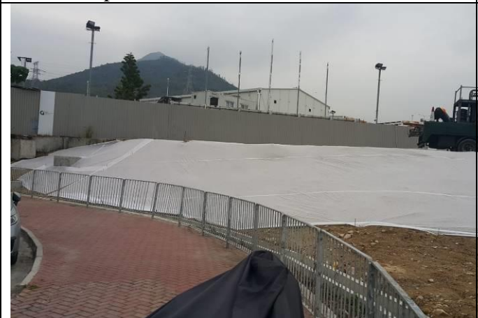
Photo 3 Hydro seeding for the exposed slope at Platform 10.
