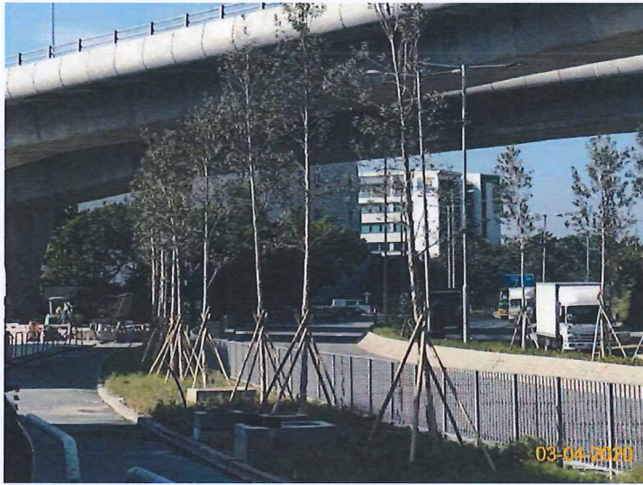
Item 3. Landscape works was commenced.
