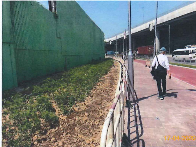
Item 3. Landscape works was commenced.
