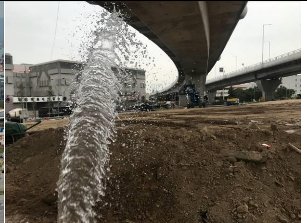
Photo 2 Water spraying by worker for un-accessible area.
