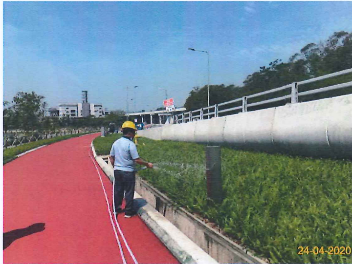
Item 3. Landscape works was commenced.
