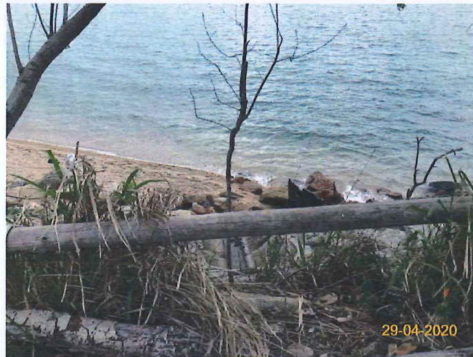
Item 7. Ensure no run-off into water body.(Outfall 1)
