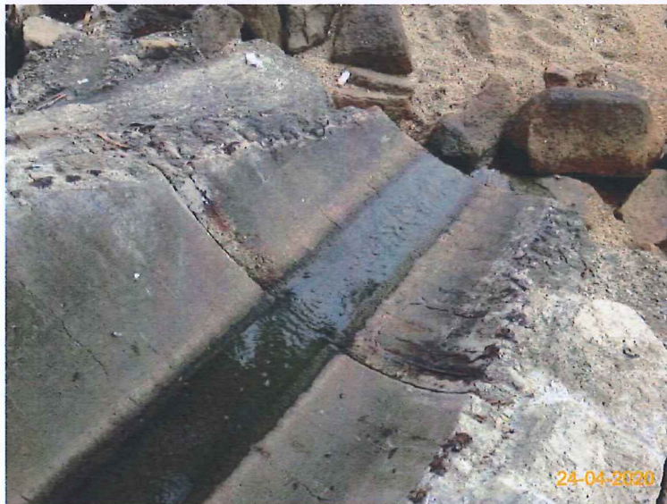
Item 7. Ensure no run-off into water body.(Outfall 1)
