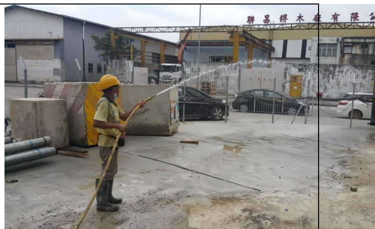
Photo 8 During the joint site inspection on 14 April 2020 water spraying had been provided for the exposed area to reduce dust impact.
