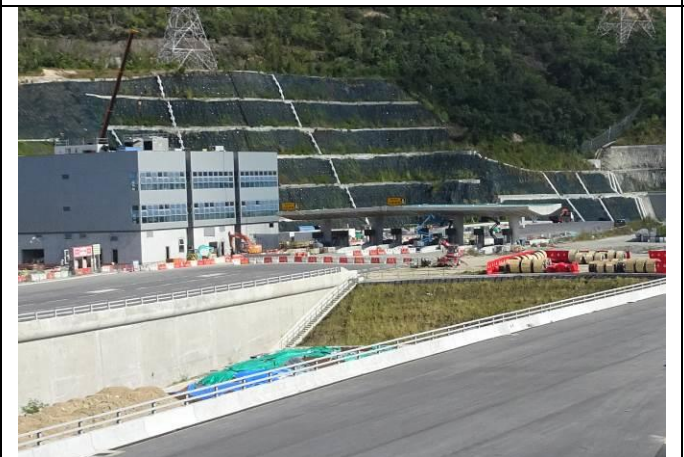
Photo 5 Hydro seeding for the exposed slope at Platform 19.
