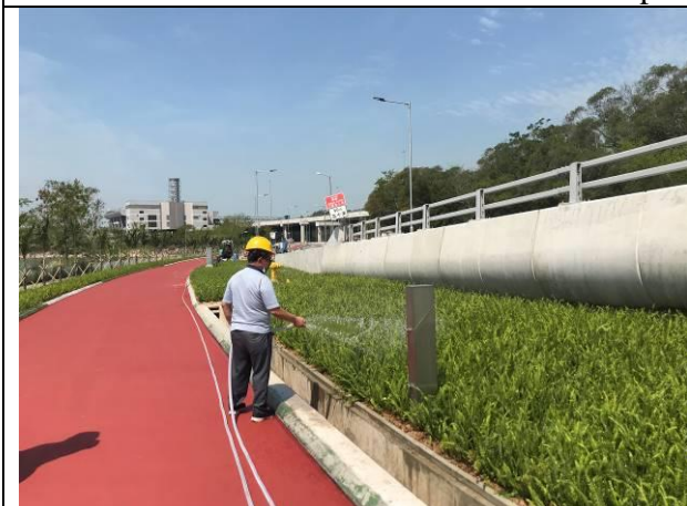
Photo 11 Planting works at Lung Mun Road
