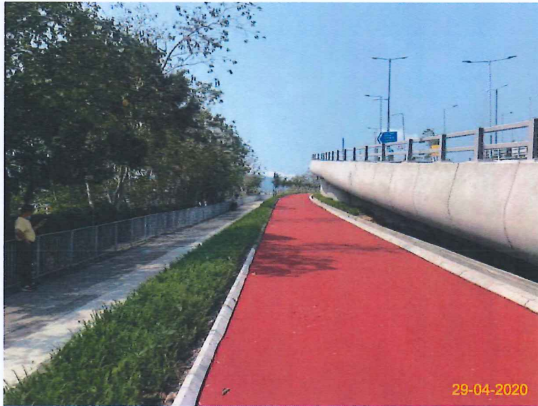
Item 3. Landscape works was commenced.
