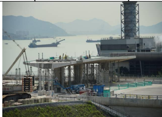
Photo 10 Modification Works at Toll Booth Area
