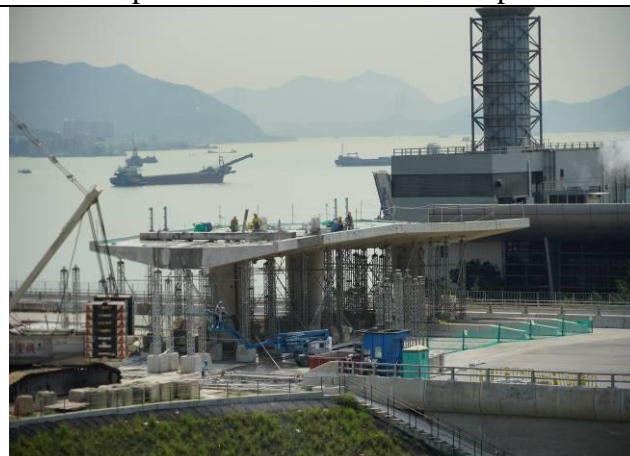
Photo 10 Modification Works at Toll Booth Area
