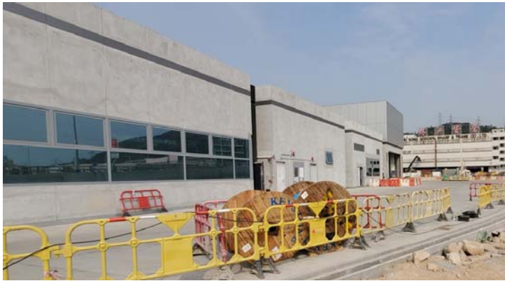
Photo 2 - Construction works at Maintenance Depot
