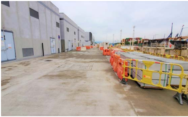
Photo 1 - Construction works at Administration Building
