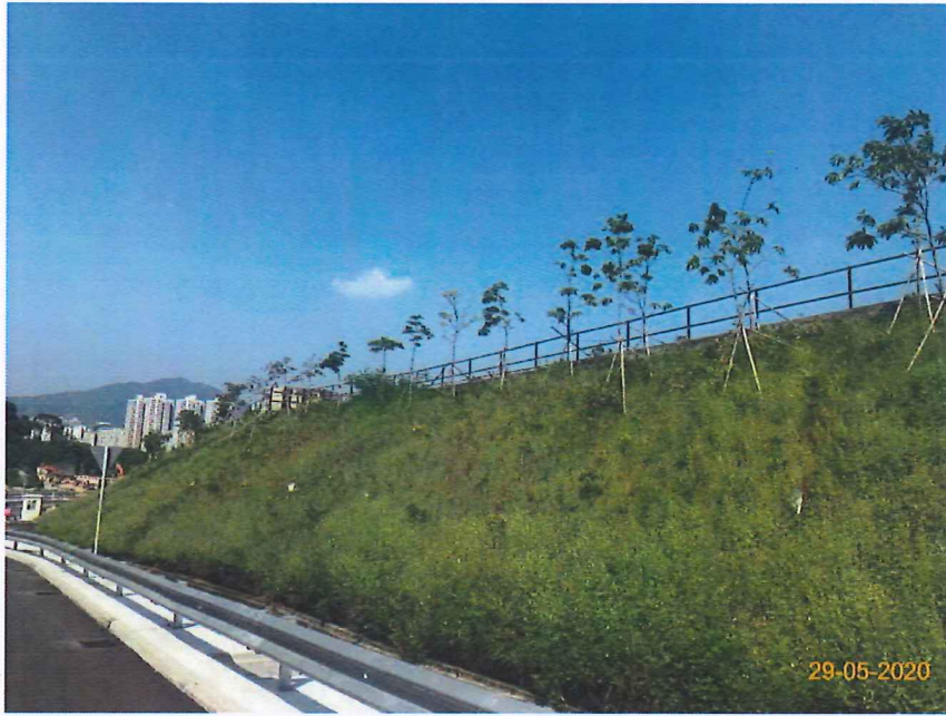
Item 3. Landscape works was commenced.
