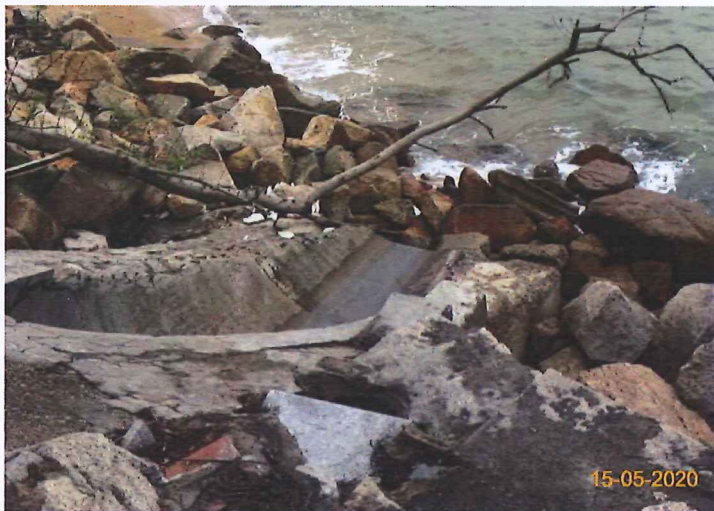
Item 7. Ensure no run-off into water body.(Outfall 1)
