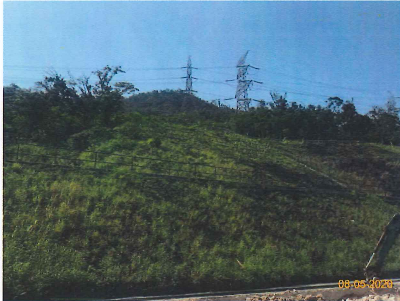
Item 3. Landscape works was commenced.
