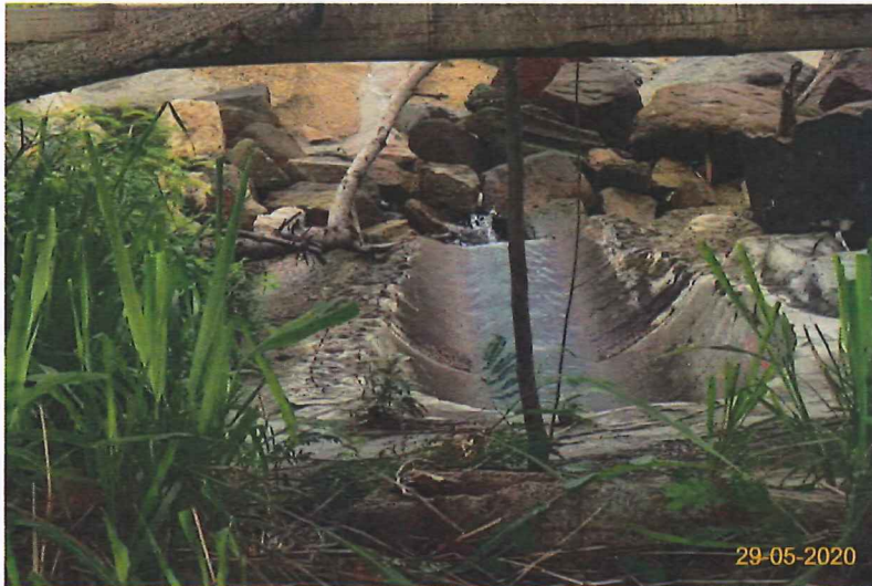
Item 7. Ensure no run-off into water body.(Outfall 1)
