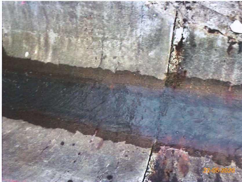
Item 7. Ensure no run-off into water body.(Outfall 1)
