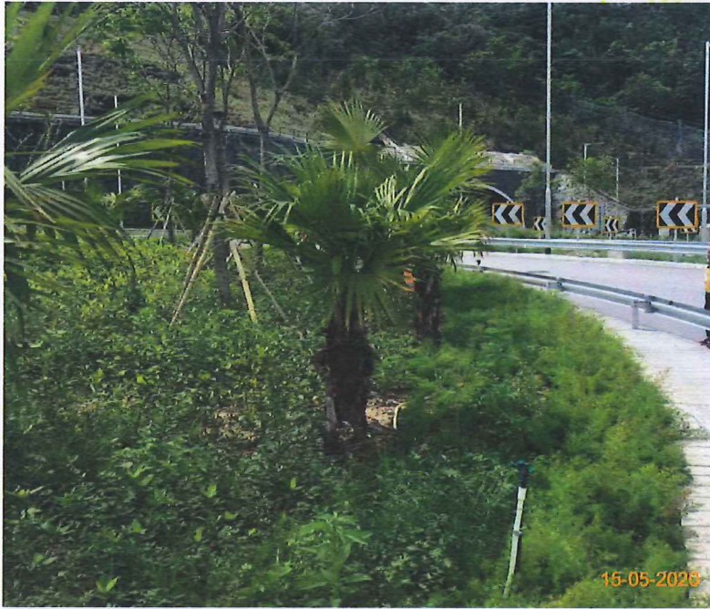
Item 3. Landscape works was commenced.
