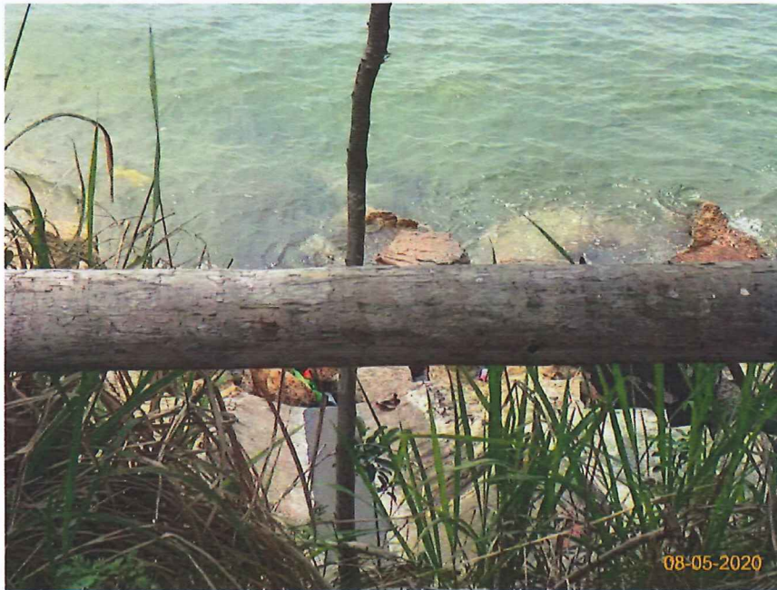
Item 7. Ensure no run-off into water body.(Outfall 1)
