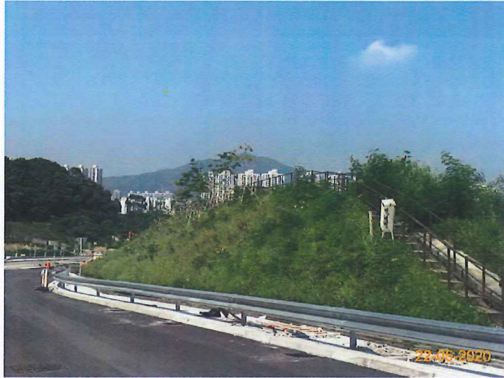
Item 3. Landscape works was commenced.
