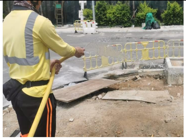
Photo 2 Water spraying by worker for un-accessible area.
