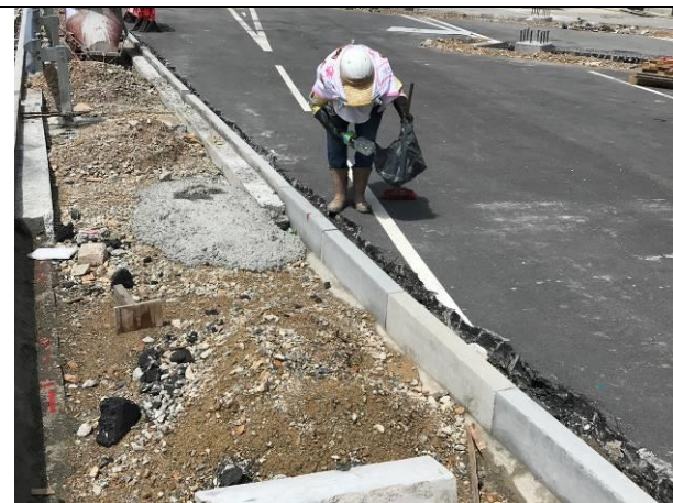
Photo 12 Housekeeping works at Toll Booth Area
