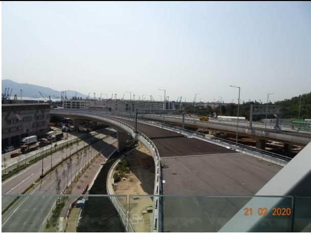
Photo 13 Most of the site area were hard paved
