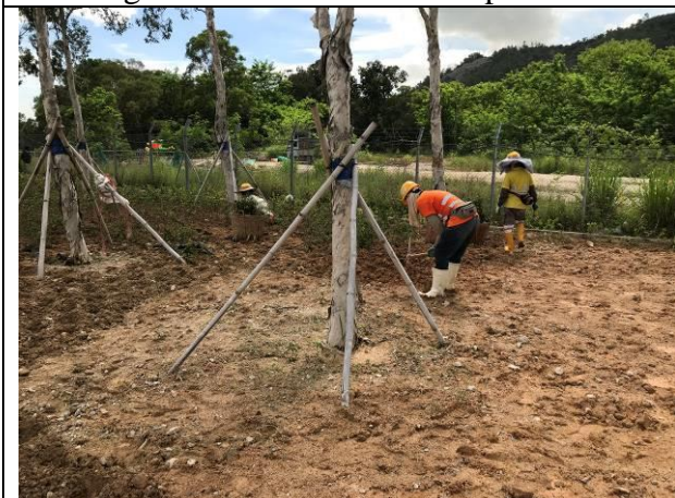
Photo 11 Landscape works at +19 Platform
