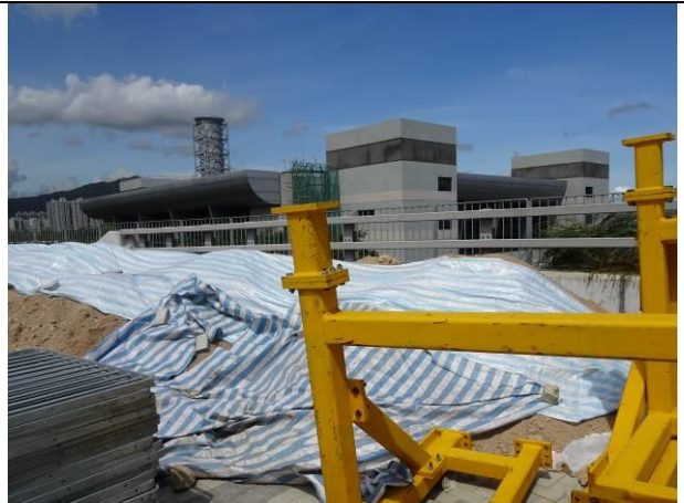
Photo 4 Covered stockpile by tarpaulin sheet.
