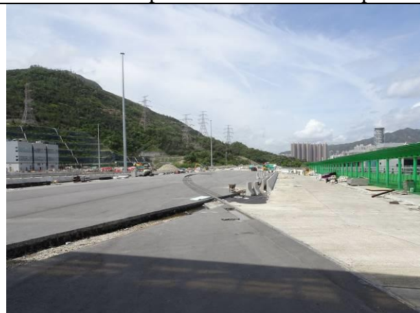
Photo 10 Site Area near the ASR6 were hard paved
