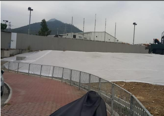
Photo 3 Hydro seeding for the exposed slope at Platform 10.
