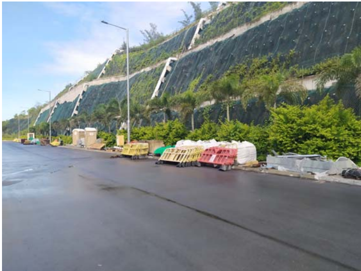
Photo 2 - Work Area nearby Main Control Building
