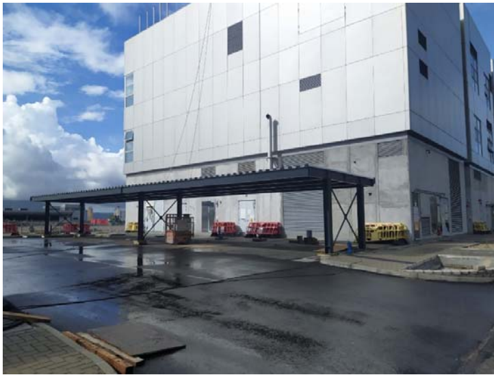
Photo 1 - Construction works at Main Control Building
