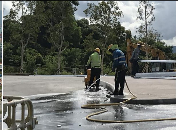
Photo 2 Water spraying by worker for un-accessible area.
