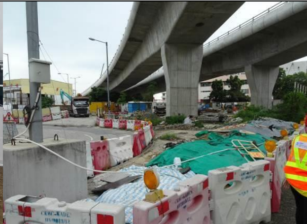
Photo 4 Covered stockpile by tarpaulin sheet.
