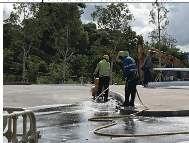
Photo 10 Remedial works at Toll Booth Area
