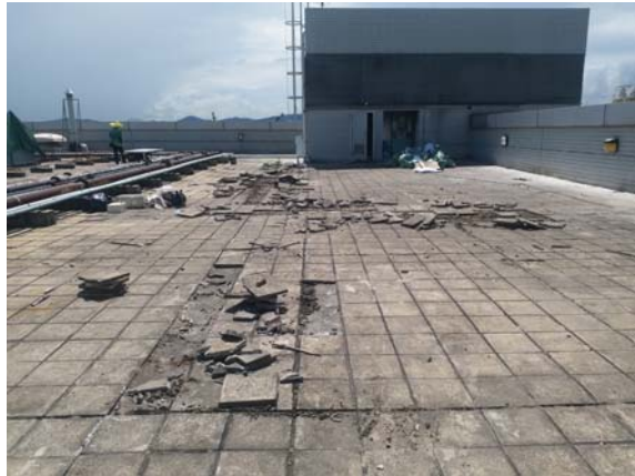
Photo 1 & 2 - Renovation works were undertaken by other contract nearby ASR6
