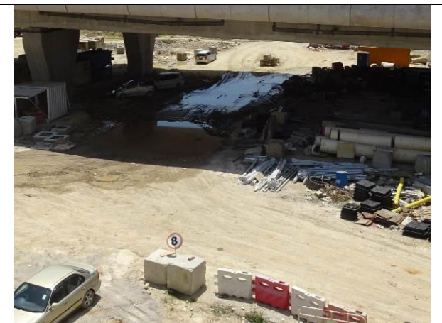
Photo 6 All vehicles using the haul road had enhanced to control the speed below 8km/hr to reduce dust emission.
