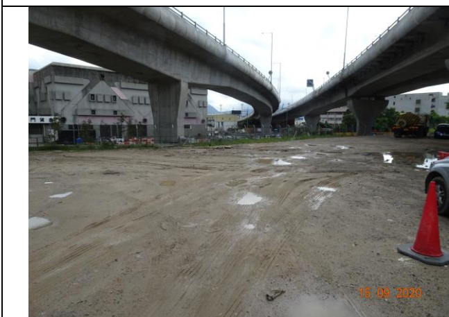
Photo 9 During the joint site inspection on 15 September 2020 water spraying had been provided for the exposed area to reduce dust impact.
