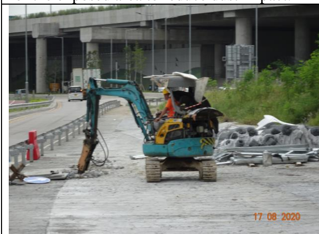
Photo 11 Remedial works at Portion H
