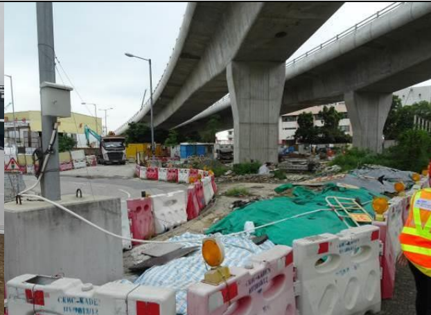
Photo 4 Covered stockpile by tarpaulin sheet.
