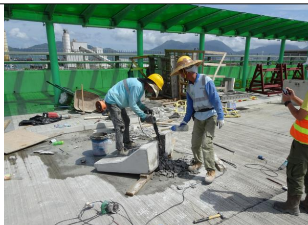
Photo 8 During the joint site inspection on 8 September 2020 water spraying had been provided for the breaking works to reduce dust impact.
