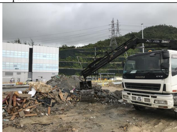
Photo 10 Housekeeping works at Toll Collector Subway Area
