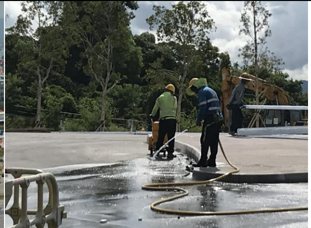
Photo 2 Water spraying by worker for un-accessible area.
