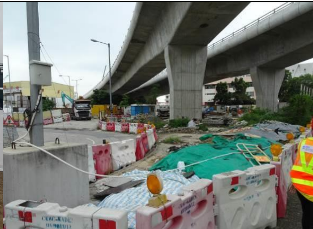
Photo 4 Covered stockpile by tarpaulin sheet.
