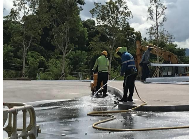
Photo 2 Water spraying by worker for un-accessible area.
