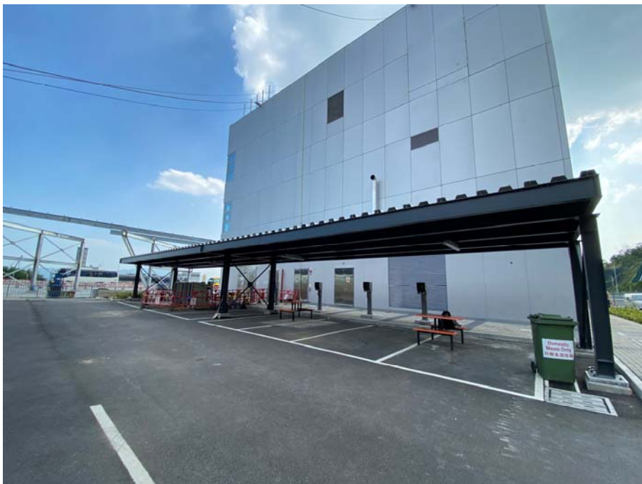
Photo 2 - Main Control Building
