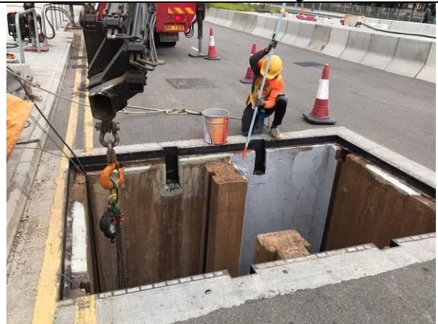
Photo 10 Remedial works at Portion H
