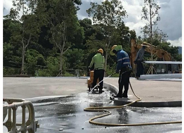
Photo 2 Water spraying by worker for construction activities.
