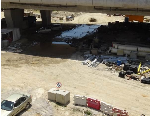
Photo 7 All vehicles using the haul road had enhanced to control the speed below 8km/hr to reduce dust emission.
