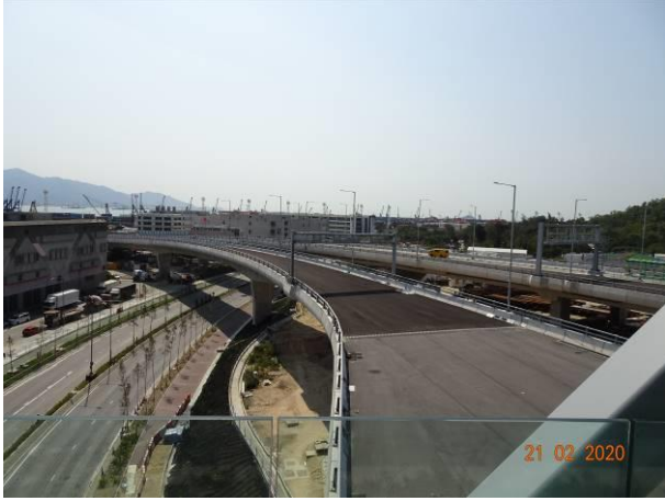
Photo 13 All of the site area under the contract were hard paved
