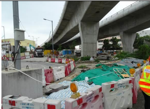
Photo 4 Covered stockpile by tarpaulin sheet.
