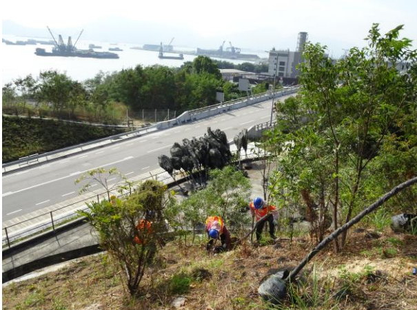
Photo 11 Remedial works at Lung Mun Road
