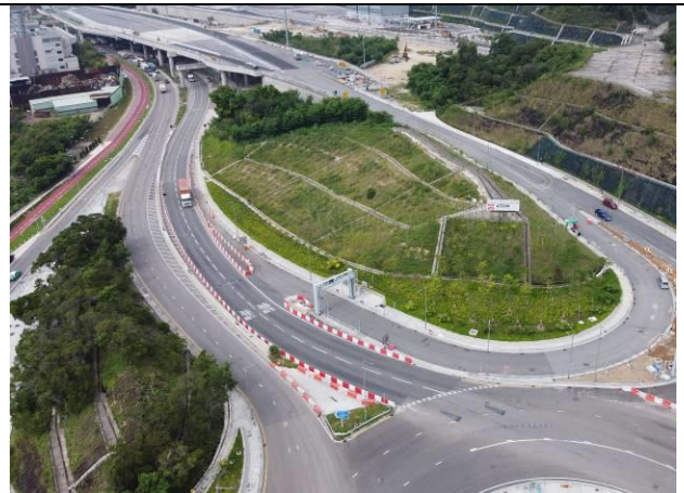
Photo 12 Most of the site area were hard paved
