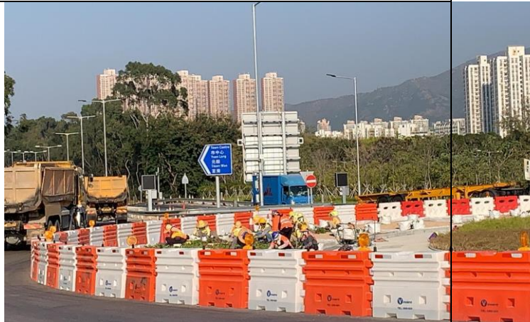
Photo 10 Remedial works at Roundabout
