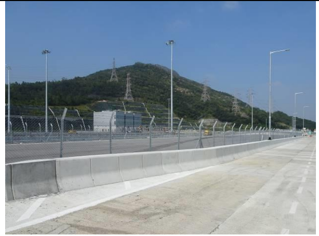
Photo 8 During the joint site inspection on 27 October 2020, no dusty activities were observed from the site near the monitoring station.
