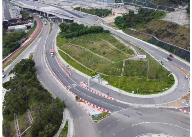
Photo 12 All of the site area under the contract were hard paved
