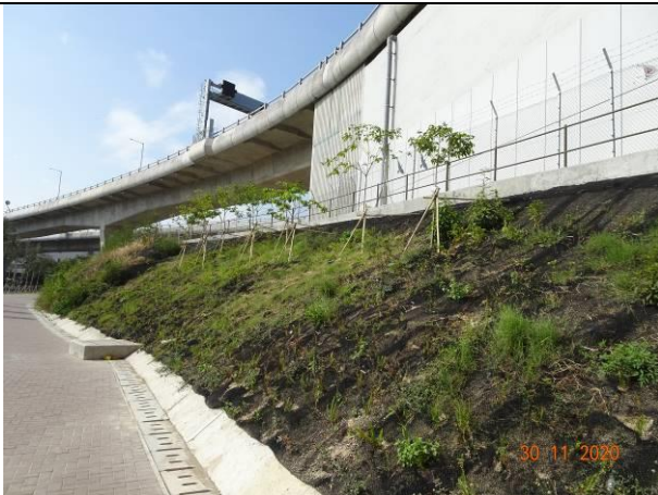
Photo 3 Hydro seeding for the exposed slope at Platform 10.
