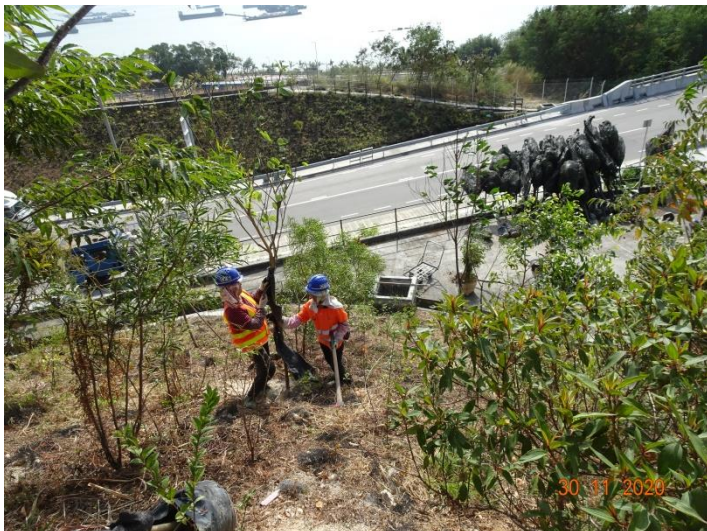
Replacement works for poor health tree
