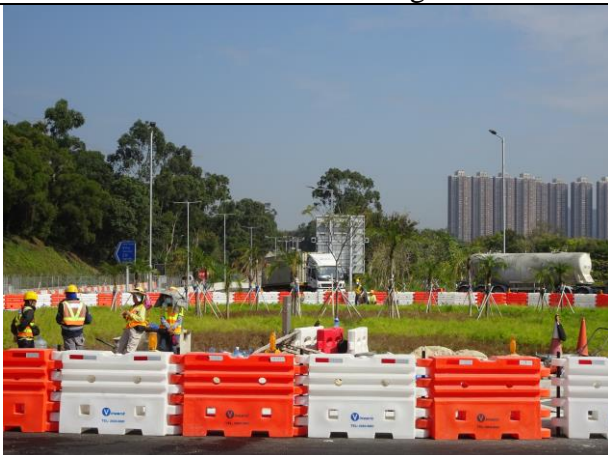
Photo 11 Remedial works at Roundabout
