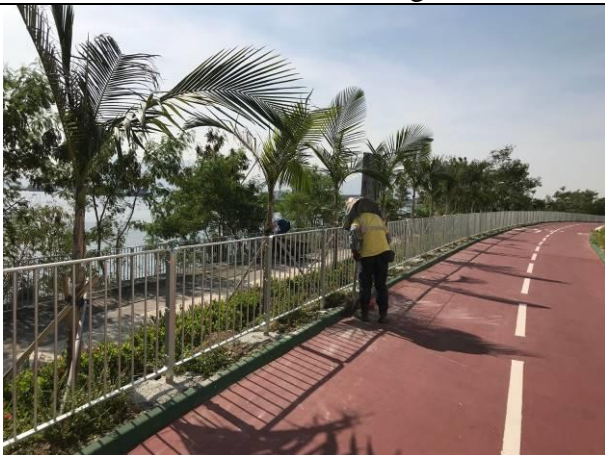
Photo 11 Remedial works at Portion H
