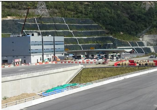
Photo 5 Hydro seeding for the exposed slope at Platform 19.
