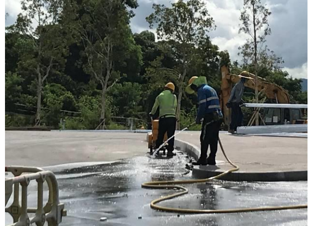
Photo 2 Water spraying by worker for construction activities.
