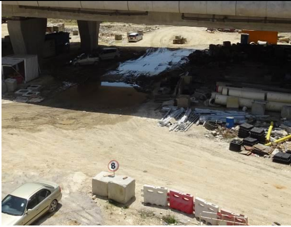
Photo 7 All vehicles using the haul road had enhanced to control the speed below 8km/hr to reduce dust emission.
