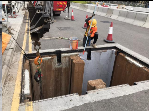
Photo 10 Remedial works at Lung Mun Road
