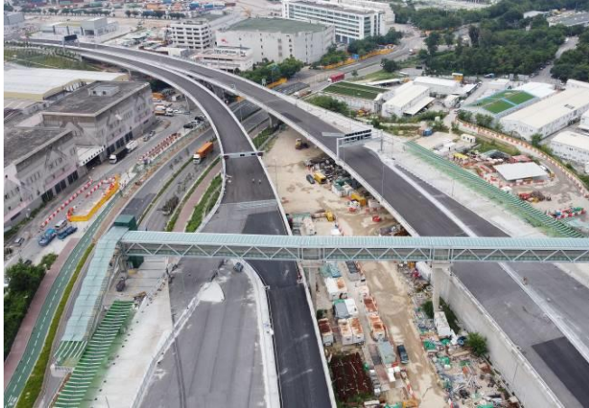
Photo 1 All access road within the Contract had been hard paved
