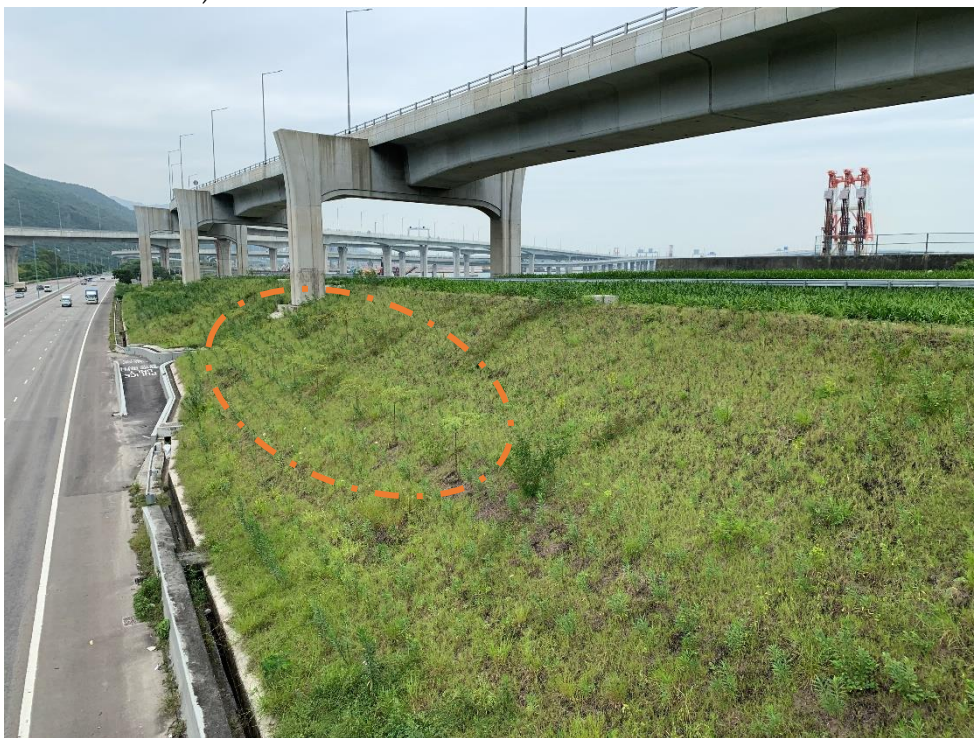
Photo 52: Bombax ceiba on Slope 10NW-C/FR17 within Zone 3 (Taken on: 8 October 2020)
