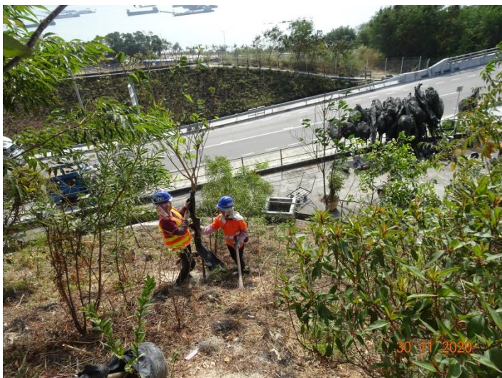
Replacement works for poor health tree
