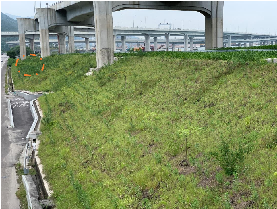
Photo 51: Bombax ceiba on Slope 10NW-C/FR17 within Zone 3 (Taken on: 8 October 2020)
