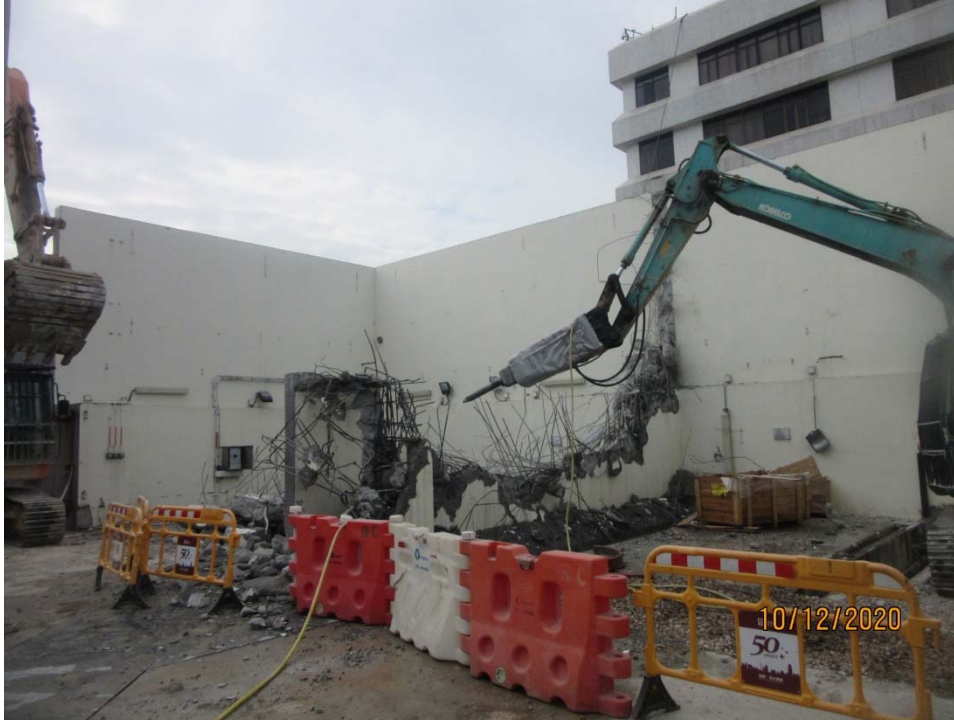
Photo 1 - Water spraying was applied during rock/cement breaking to prevent dust
