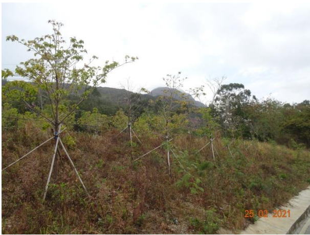
General View for Slope 5SE-D/C215
