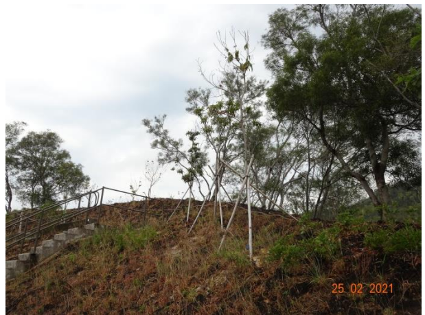
General View for Slope 5SE-D/C21
