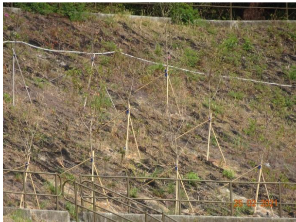
General View for Slope TP_A
