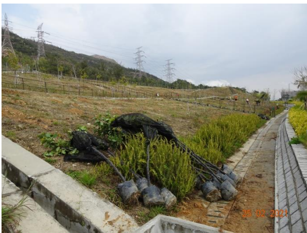
Tree re-planting works was conducted at slope 5SE-D/C170
