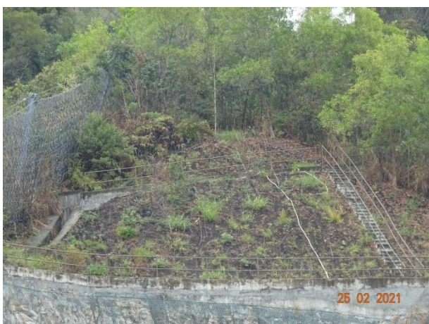
General View for Slope TP_D
