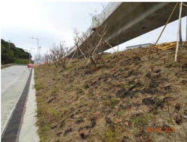
General View for Zone 1B
