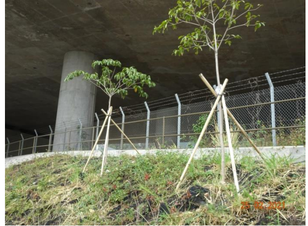
General View for Slope 5SE-D/C18
