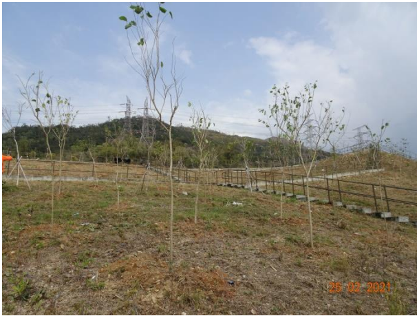
General View for Slope 5SE-D/C170
