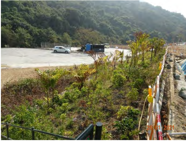
General View for Zone 1B
