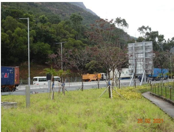
General View for Roundabout Area
