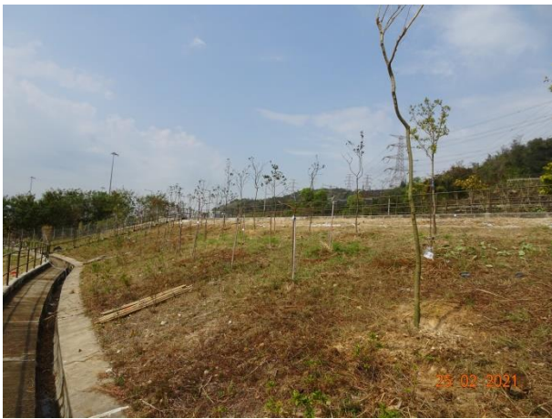
General View for Slope 5SE-D/C170
