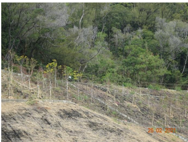
General View for Slope TP_A
