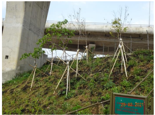
General View for Slope 5SE-D/C16
