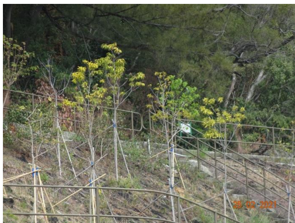
General View for Slope TP_A
