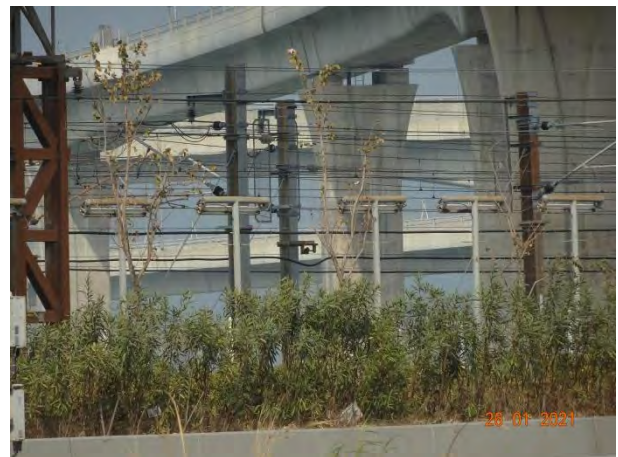
General View for Zone 3B
