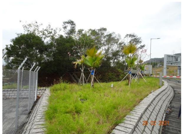
General View for Roundabout Area
