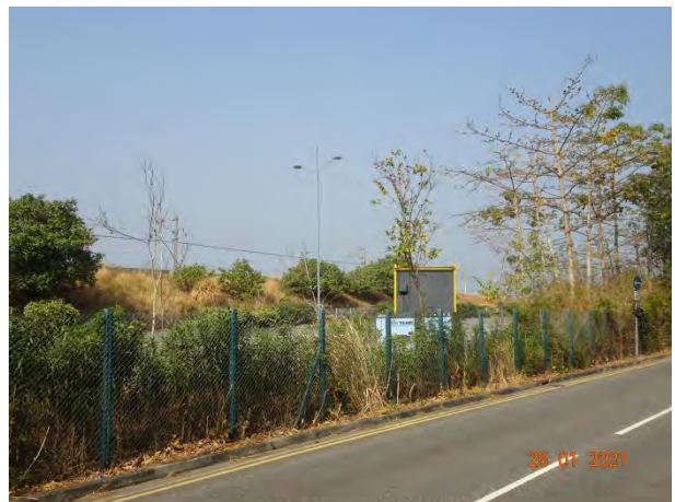
General View for Zone 3F
