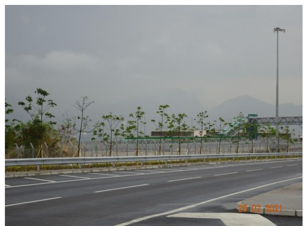
General View for Toe Planter
