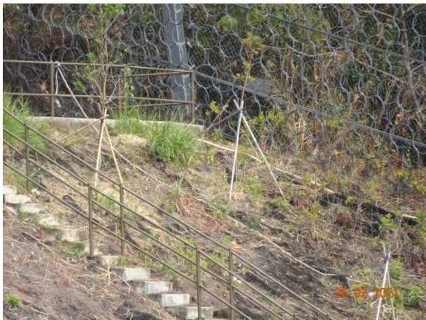
General View for Slope TP_A
