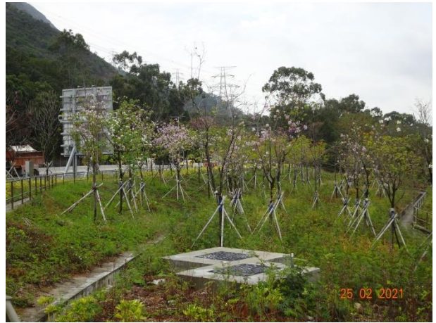
General View for Slope 5SE-D/C215
