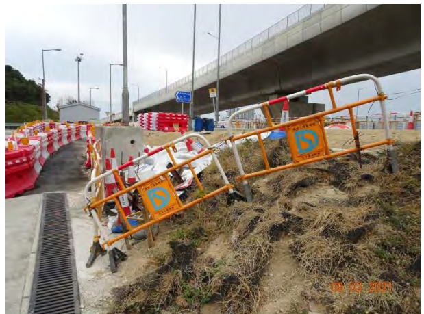
General View for Zone 1B
