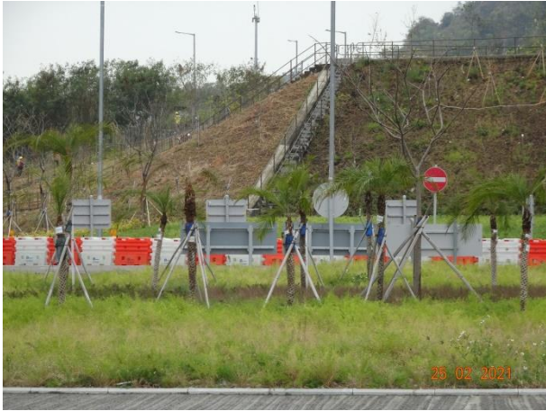
General View for Roundabout Area
