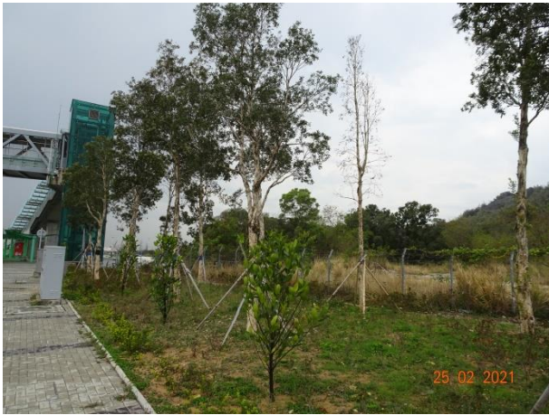
General View for Toll Plaza
