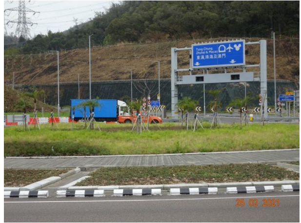
General View for Roundabout Area
