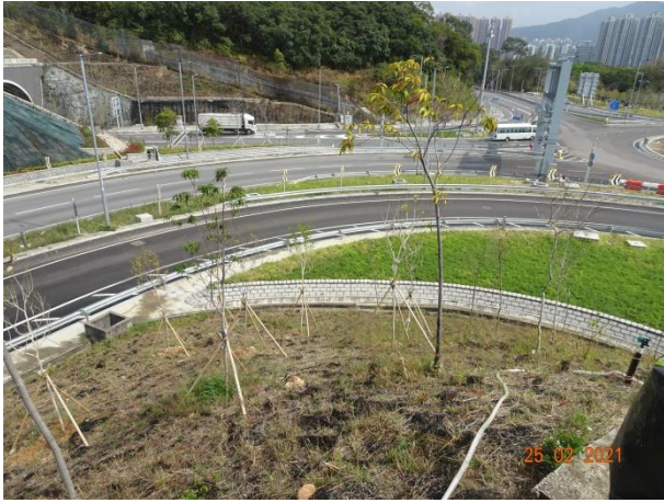
General View for Slope TP_C
