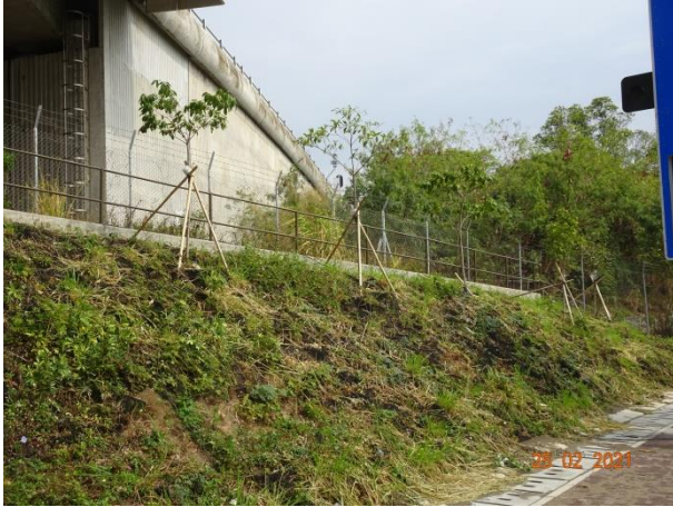
General View for Slope 5SE-D/C18
