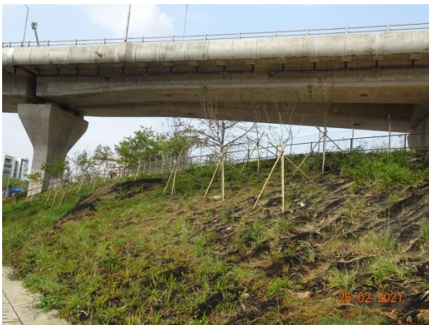
General View for Slope 5SE-D/C16
