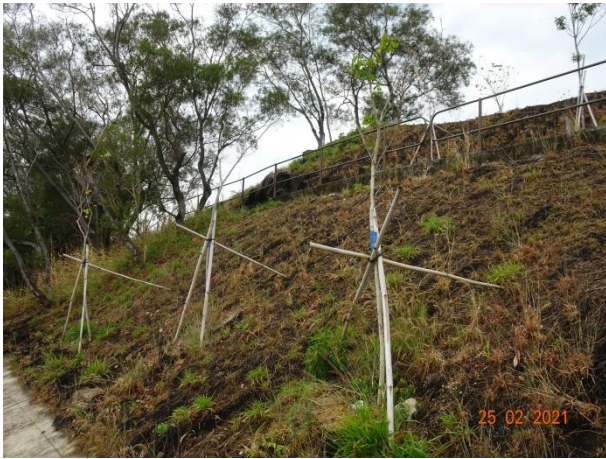
General View for Slope 5SE-D/C21
