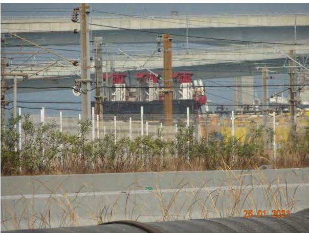
General View for Zone 3B
