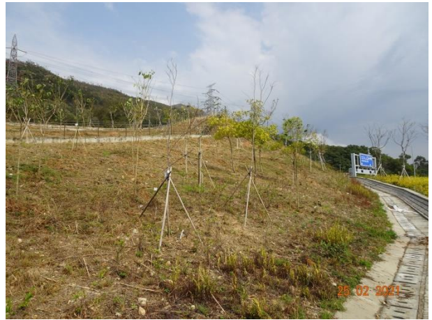
General View for Slope 5SE-D/C170
