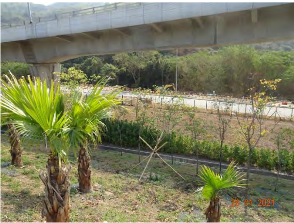
General View for Zone 3E
