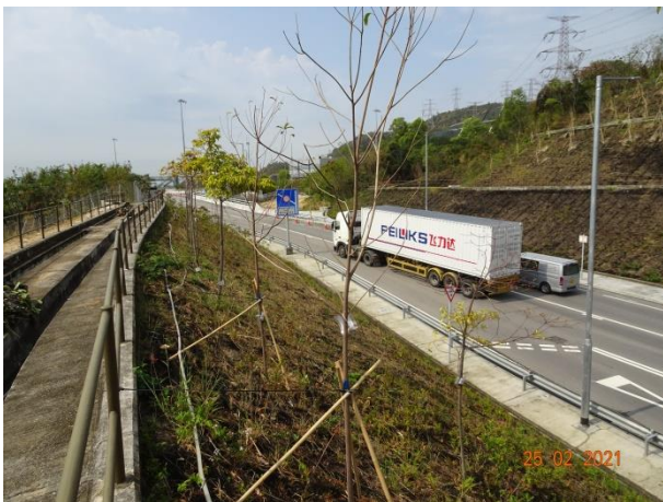
General View for Slope TP_C
