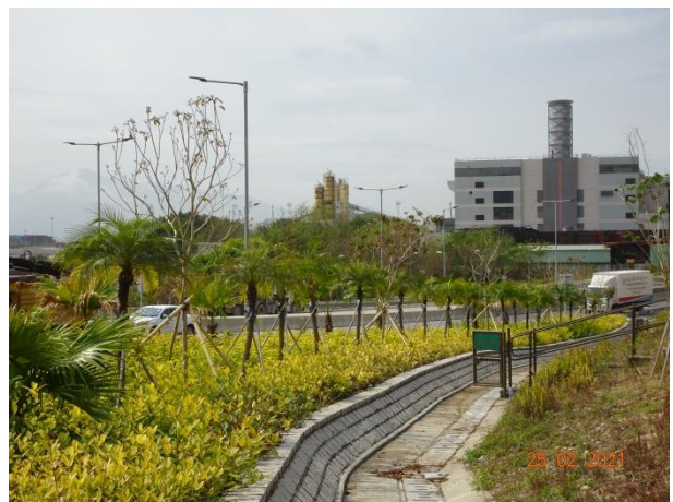
General View for Roundabout Area
