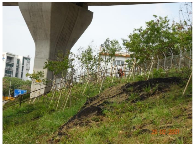
General View for Slope 5SE-D/C16
