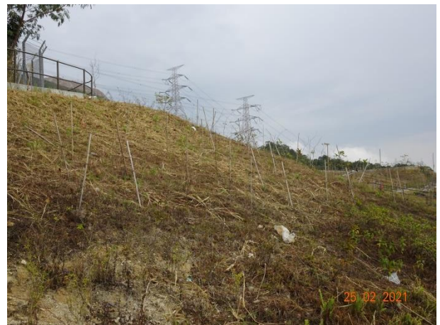
General View for Slope 5SE-D/C170
