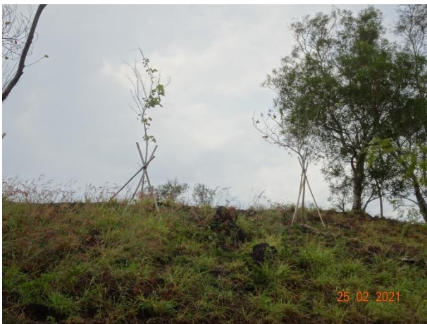
General View for Slope 5SE-D/C171
