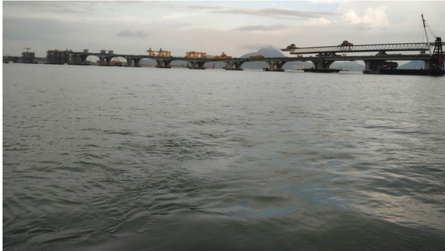
Photo 11 - Mid-Flood at IS8 on 22 September 2017
