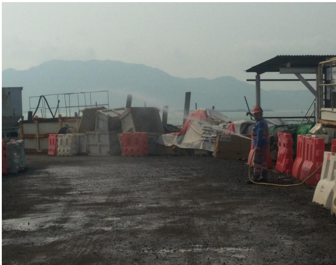
Water spraying was applied frequently on site. (Works Area Portion N-C)
