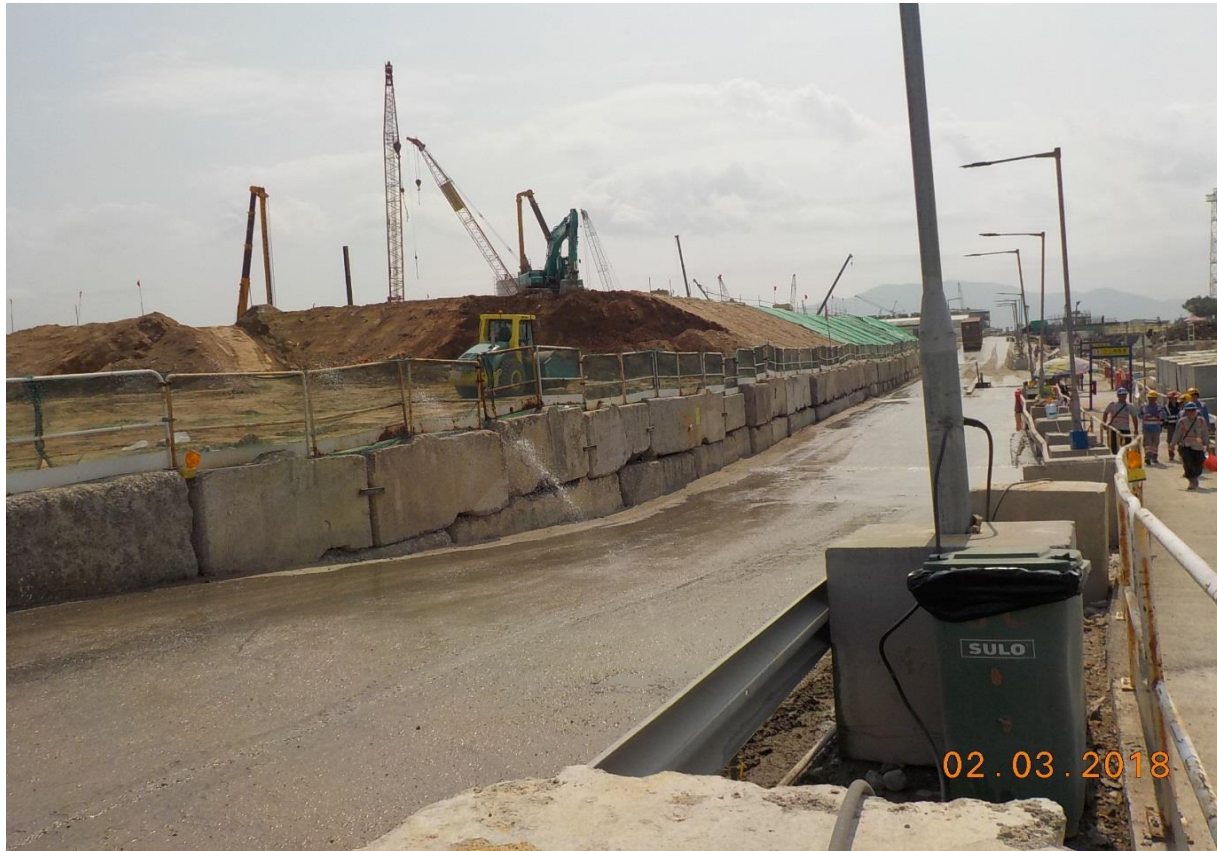
Water spraying was applied frequently on site. (Works Area Portion N-A)
