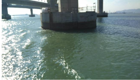
Photo 6 - Mid-Flood at SR4a on 8 August 2018
