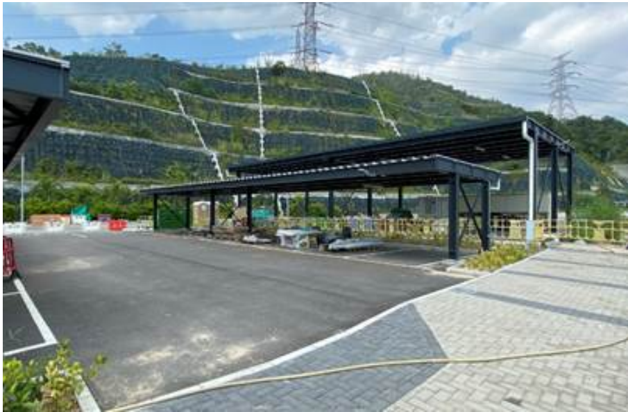
Photo 2 - Main Control Building
