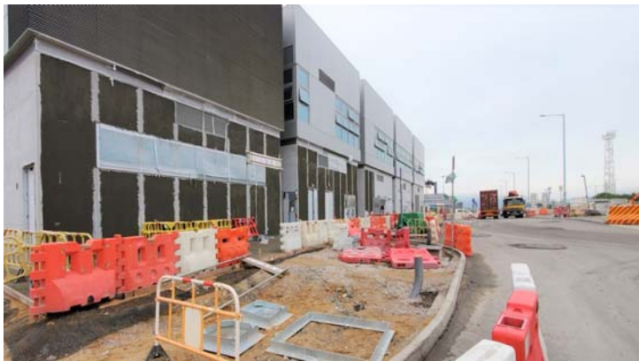
Photo 2 - Construction works at Maintenance Depot
