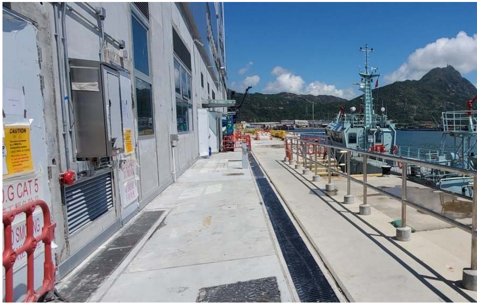
Photo 1 - Fire Services Department Building & Customs and Excise Department Building
