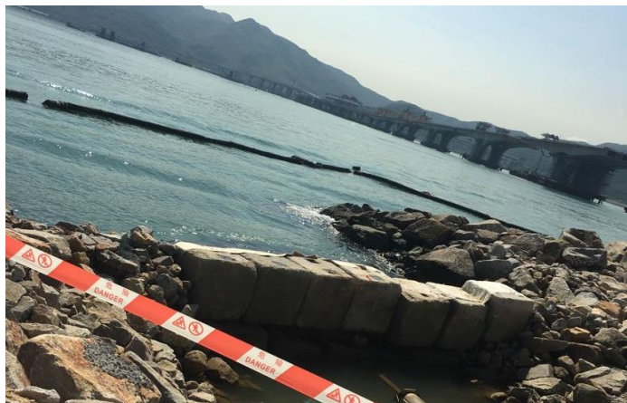
Photo record shows condition of silt curtain and active works area at outfall area on 28 September 2017.
