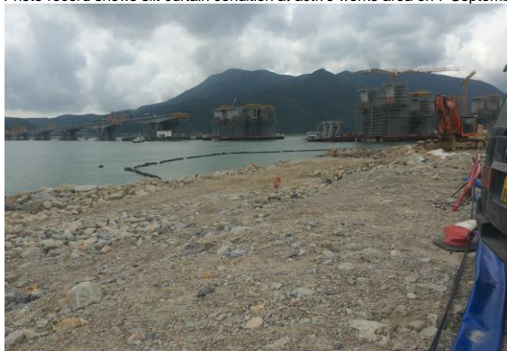
Photo record shows silt curtain condition at active works area on 14 September 2017.
