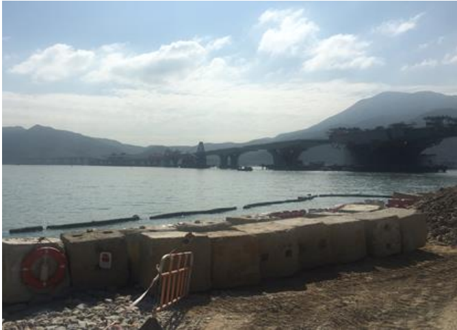
Photo record show silt curtain condition and active seawall construction area on 9 Nov 2017.
