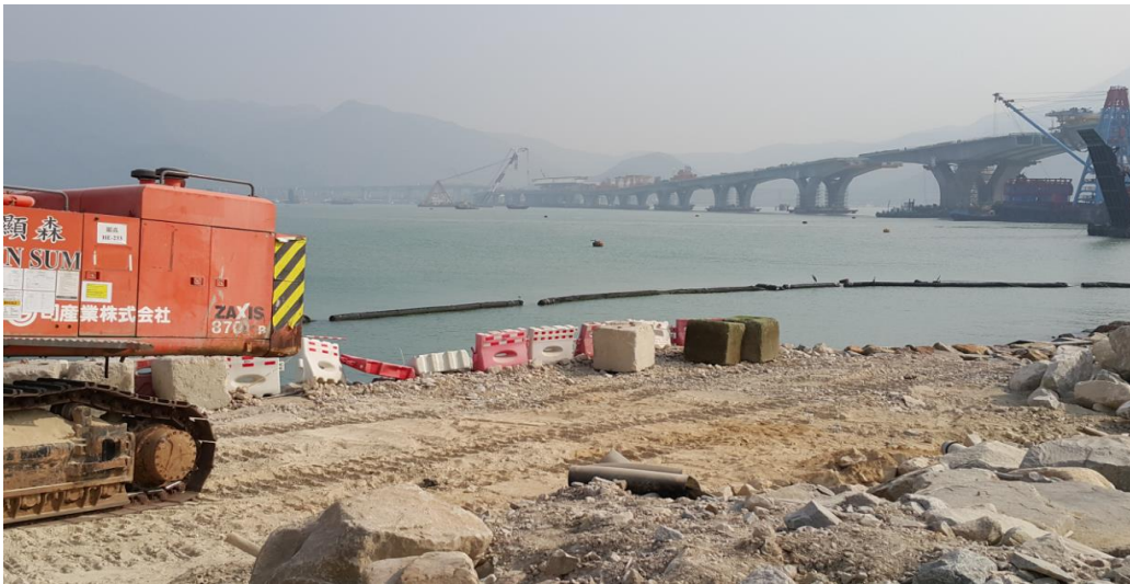
Photo record show silt curtain condition and active seawall construction area on 6 Dec 2017.
