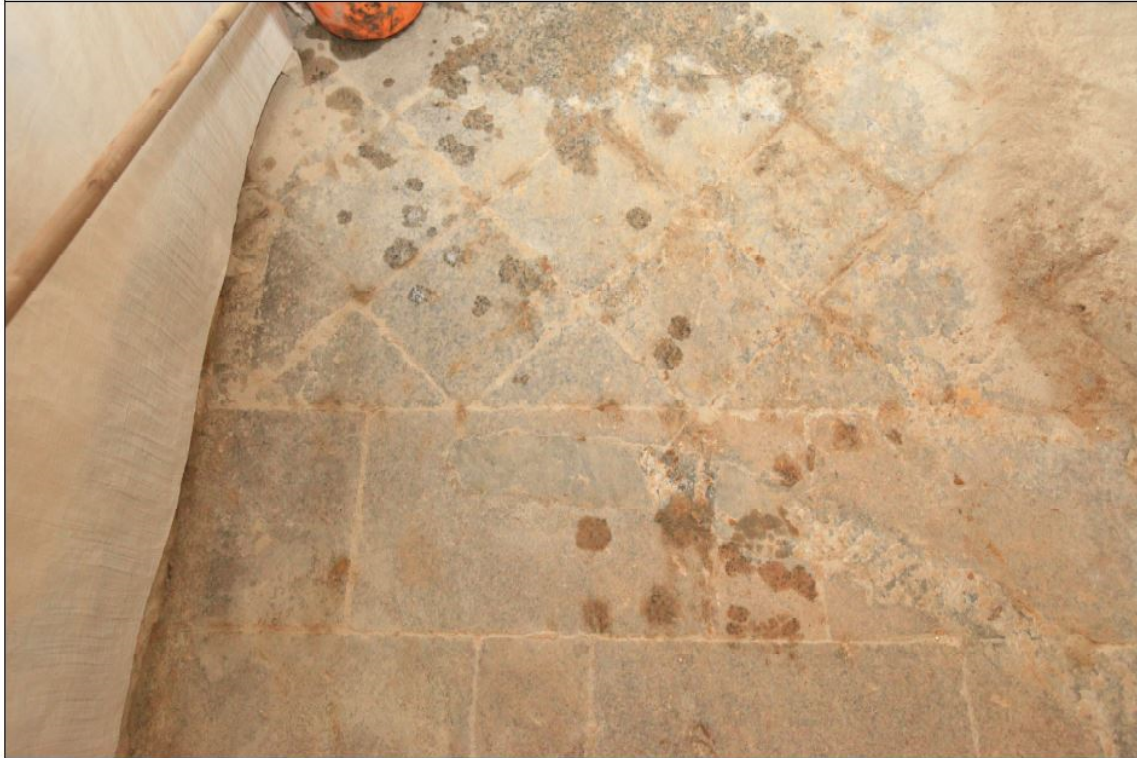
Photograph taken on 22 nd August 2013 by the Management Contractor, showing the granite border at the west archway.
