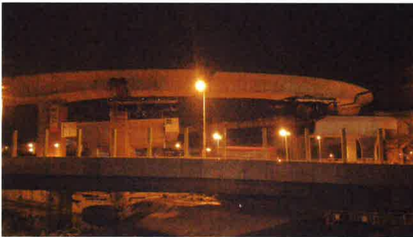
Noise from traffic in the highway, occasionally dogs barking from village
