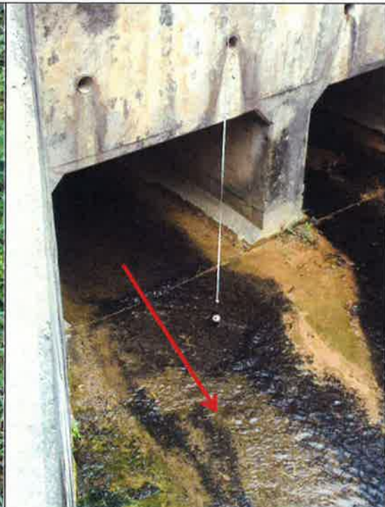
Photo 3 View of downstream of Location WM2B The water depth is approximately 0.01-0.02m.
