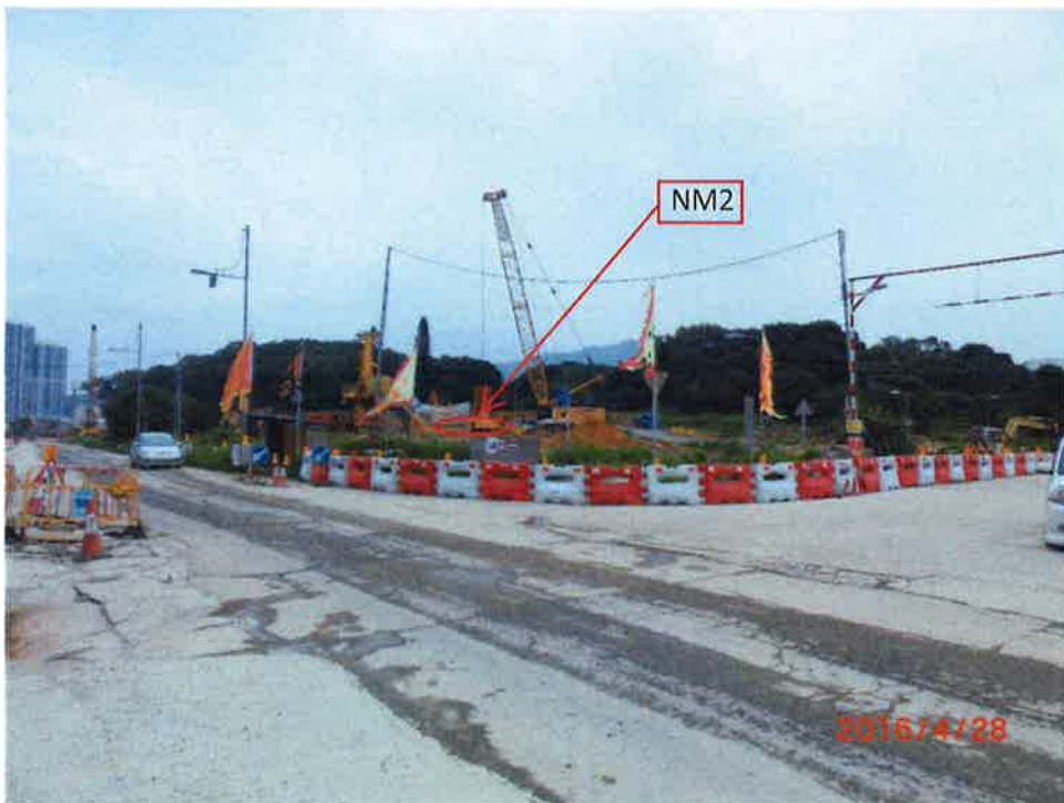
View from NM2a to the construction site
