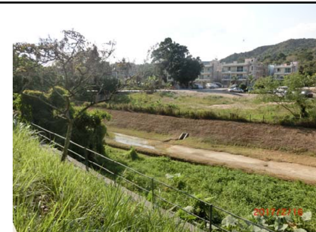
Photo 6 During site inspection on 16 February 2017 at downstream of WM3x of Ng Tung River, it was observed that turbid water was flowing from an outfall and the source of turbid water was come from the adjacent village.
