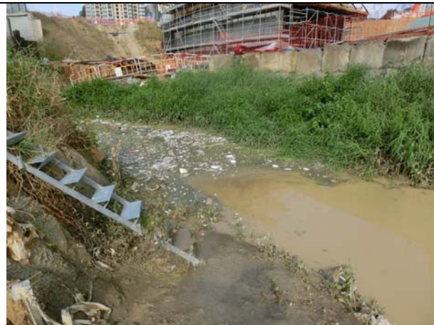
Photo 3 On 22 February 2017, muddy water and cumulated rubbish was observed at WM1 after rain.
