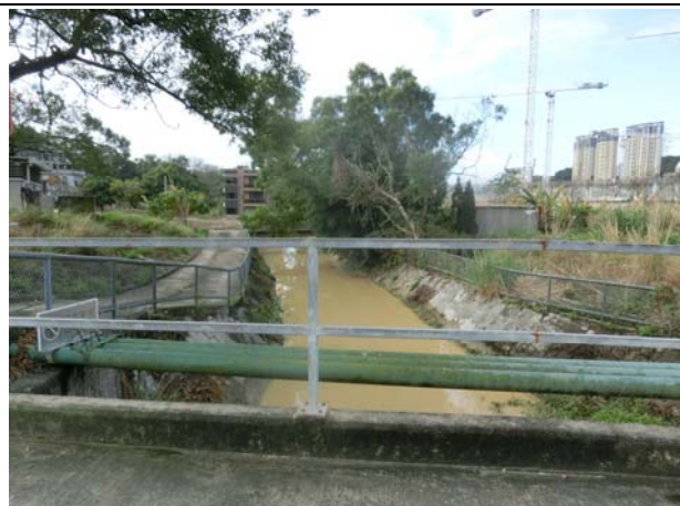
Photo 4 On 22 February 2017, muddy water was observed at WM1-C after rain.
