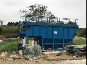
**Photo 8** Wastewater treatment facilites were provided for Bridge D.
