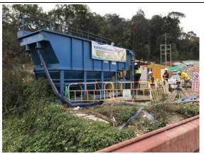
**Photo 11**A wastewater treatment facility with AquaSed SH-20 was implemented.
