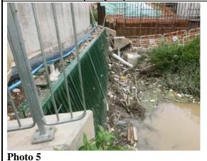
As observed during site inspection in early May 2017, since large amount of rubbish was cumulated near at the water gate near WM1, the muddy water generated under rain was stagnant and could not flow to downstream.
