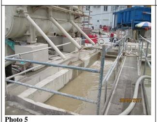
During weekly site inspection at South Portal by ET in April 2017, it was observed the wastewater treatment facility implemented on site was function properly and the treated water to be discharged was clear.
