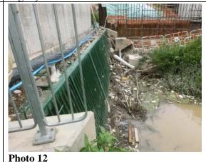
As observed during site inspection on 18 and 24 May 2017, since large amount of rubbish was cumulated near at the water gate near WM1, the muddy water generated under rain was stagnant and could not flow to downstream.
