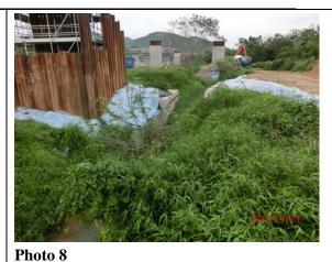
The slope adjacent to river course was covered with tarpaulin sheet to minimize muddy runoff. Moreover, concrete block as temporary bund was provided align the river course and no turbid runoff and discharge was made from the site.
