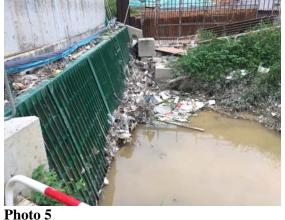
As observed during site inspection on 25 May 2017, since large amount of rubbish was cumulated near at the water gate near WM1, the muddy water generated under rain was stagnant and could not flow to downstream.
