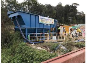
**Photo 5**Wastewater treatment facility with AquaSed SH-20 was implemented.
