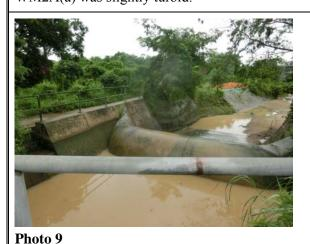
On 19 June 2017, it was observed that the nylon dam was deflated and muddy water was flowing to downstream.
