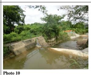
On 22 June 2017, it was observed that the nylon dam was deflated and muddy water was flowing to downstream.
