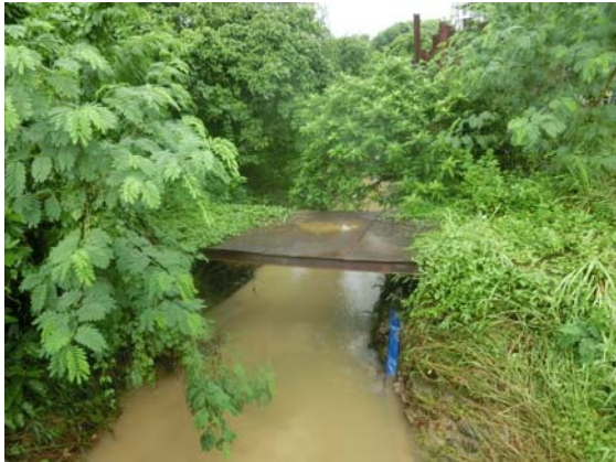
Photo 1 On 24 July 2017, muddy water was observed at WM2A(a).
