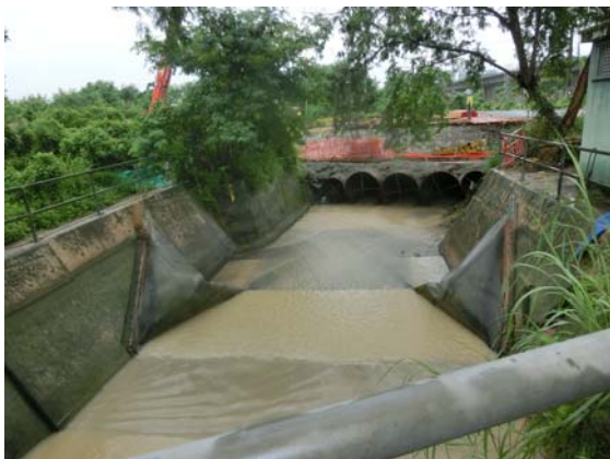
Photo 5 On 24 July 2017, it was observed that the nylon dam was deflated and muddy water was flowing to downstream.
