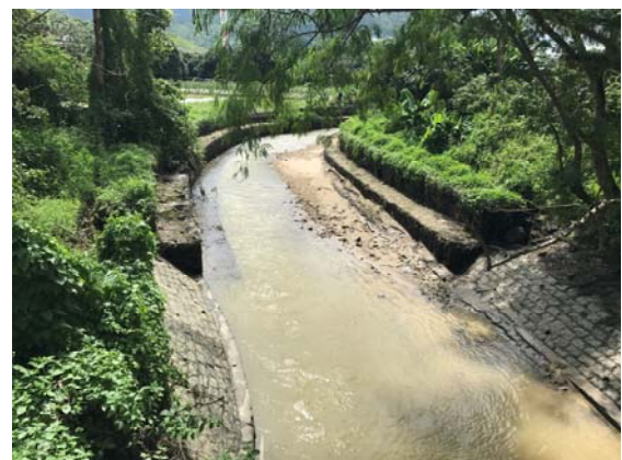
Photo 6 On 24 July 2017, loose sediment was observed at river bed after nylon dam deflated.
