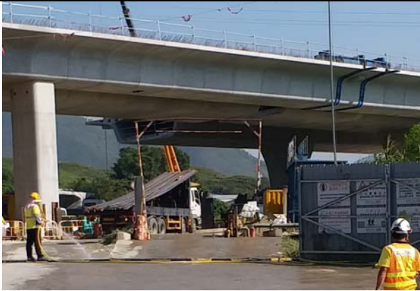
Photo 7 (Bridge D Site Exit under LT/C6)
