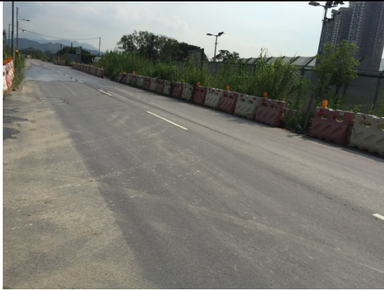
Photo 7 (Bridge D (D08))
