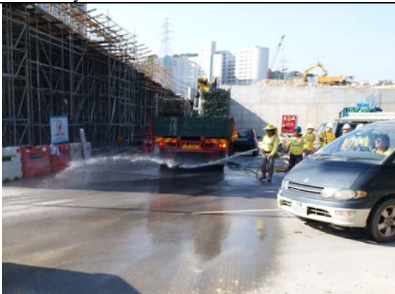
Photo 11 (Bridge Y Site Exit under LT/C6)
