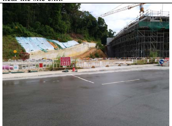
Photo 18 (opposite to Bridge Y)
