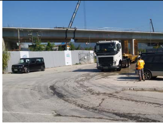
Photo 8 (Bridge D Site Exit under LT/C6)
