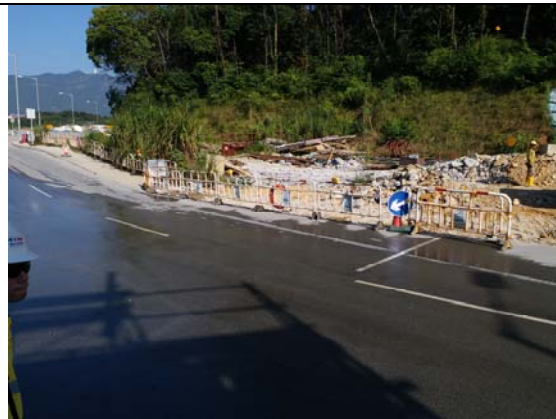
Photo 12 (Bridge Y Site Exit under LT/C6)
