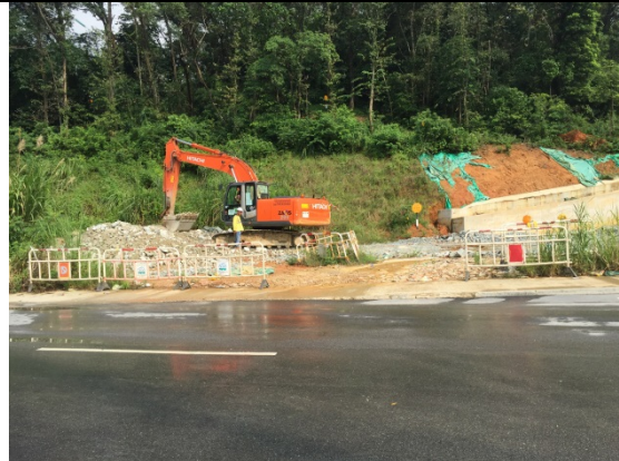
Photo 6 (opposite to Bridge Y)
