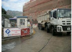
**Photo 7 (Admin Building under C2)** Wheel washing facilities was provided within the construction site and site vehicle was cleaned prior leaving the site.
