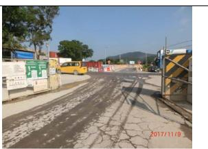
**Photo 10 (South Portal and Site office under C6)** No muddy trails and dust and soil carrying by site vehicles to public road were observed outside the site exit.
