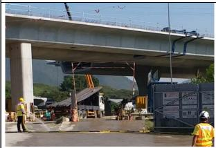
**Photo 3 (Bridge D Site Exit under LT/C6)** Wheel washing facilities were provided and properly maintained by CCKJV. A bund was provided to prevent muddy water from flowing out of the site.
