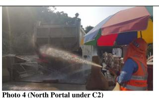
The vehicle site exit of North Portal Site Area (LT/C2) was located on STK Road. Wheel washing facilities was provided within the construction site and site vehicle was cleaned prior leaving the site.
