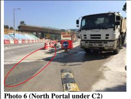
No dust and soil carrying by site vehicles to STK road were observed after wheel washing. However, mud and debris was observed at the edges of the road in the exiting STK road which suspected to be caused by frequent use of dump truck transporting loose material to NENT and the majority of dump truck was not belong to LT/HYW project.
