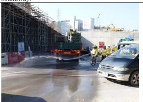
**Photo 7 (Bridge Y Site Exit under LT/C6)** Wheel washing facilities were provided and properly maintained by CCKJV. The wastewater from wheel washing was directed to AquaSed for de-silting.
