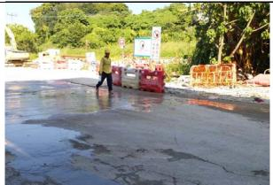
**Photo 5 (Chuk Yuen Rd Site exit under LT/C6)** Wheel washing facilities were provided and properly maintained by CCKJV. The wastewater from wheel washing was directed to catchpit for soakaway.
