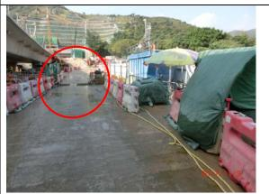
**Photo 9 (South Portal and Site office under C6)** Wheel washing facilities was provided within the construction site and site vehicle was cleaned prior leaving the site.
