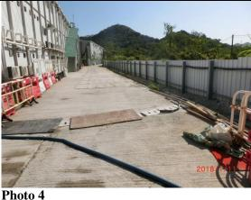
Joint site inspection was conducted on 11 January 2018. It was observed that site hoarding with sealed footing was installed and no runoff from the site area was anticipated.
