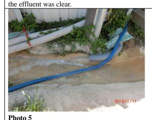
Joint site inspection was conducted on 11 January 2018. It was observed that wastewater treatment facilities were function properly for South Portal and the effluent was clear.
