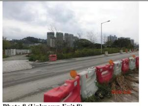
**Photo 8 (Unknown Exit 8)** The condition of unknown site exit 8 was fair but some mud and debris were found on the kerbs and middle of LMH road. The maintenance party/ ownership of the site exit is unknown.
