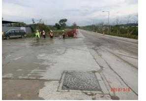
**Photo 10 (Bridge D Site Exit under LT/C6)** The condition of Bridge D Site Exit under LT/C6 and adjoined LMH road was satisfactory without mud and debris.
