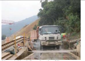
**Photo 4 (North Portal under C2)** The vehicle site exit of North Portal Site Area (LT/C2) was located on STK Road. Wheel washing was provided within the construction site to ensure all site vehicles were washed prior leaving the site.
