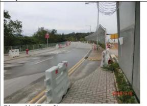
**Photo 11 (Gate 2)** Wheel washing facilities were provided for Gate 2 site exit and properly maintained by CCKJV. The condition of Gate 2 and adjoined LMH road was satisfactory without mud and debris.
