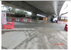
**Photo 12 (Bridge Y Site Exit under LT/C6)** Wheel washing facilities were provided for Bridge Y site exit and properly maintained by CCKJV. The condition of Bridge Y site exit and adjoined LMH road was satisfactory without mud and debris.
