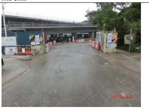
**Photo 10 (South Portal under C6)** No muddy water/ slurry was found at the site exit after the wheel washing facilities.
