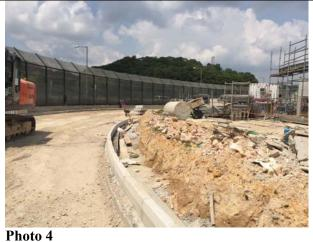
The boundary of Boundary Control Point (BCP) is surrounded by chain link fencing with concrete foot. Moreover, road kerb was constructed at the boundary of Contract SS C505 and no overflowing of site runoff was observed.
