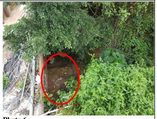
**Photo 6**During site inspection on 10 May, it was observed that the water flowing through Box Culvert BC02 was clear but trace amount of sediment / mud was observed at channel bed, which suspected to be caused by the inflow of muddy water from previous days.
