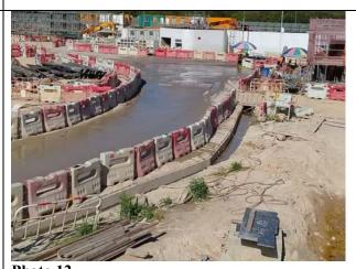
**Photo 12**Temporary drainage system was implemented to divert the wastewater to the Aquased.
