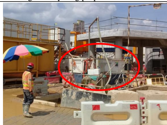
Photo 10 The wastewater treatment facilities were implemented as per the drainage plan.
