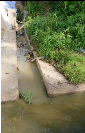
Photo 9 As reported by the Contractor of Contract 6, inflow of turbid water was occasionally observed from the open channel which receiving the stormwater from the Sha Tau Kok Road.
