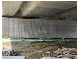
**Photo 5**Temporary bunding was provided to minimize the risk site runoff flowing into the stream.
