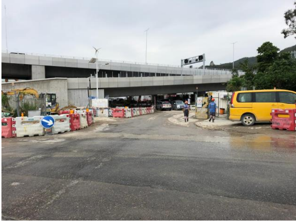
Photo 5 (Main Exit under LT/C6)
