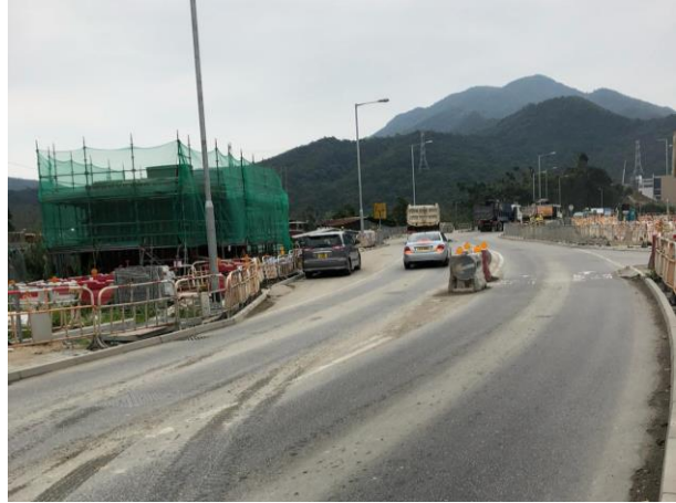
Photo 6 (Main Exit under LT/C6)
