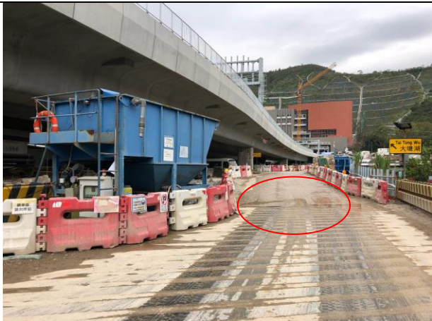
Photo 3 (Main Exit under LT/C6)
