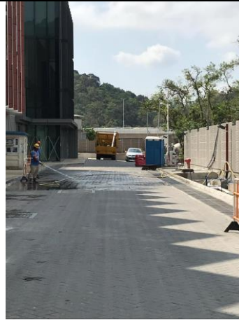
Photo 10 (Admin Building under LT /C2)
