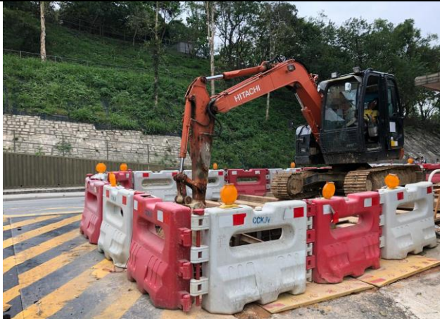
Photo 1 (temporary works area under LT/C6)
