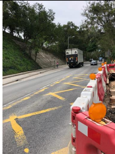
Photo 2 (temporary works area under LT/C6)
