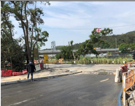
Photo 11(Admin Building under LT /C2)
