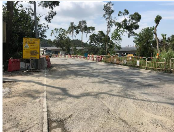
Photo 12(Admin Building under LT /C2)
