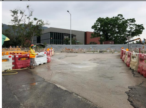
Photo 4 (Main Exit under LT/C6)
