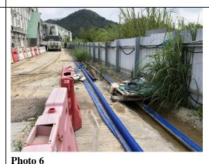
Site hoarding with footing sealed was erected at site boundary which adjacent to the stream to minimize the risk of site runoff flowing into the exiting stream.
