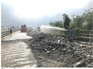
Photo 2 Wet the exposed stockpile and demolition activities in daytime.
