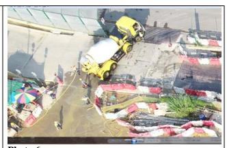
**Photo 6**Manual wheel washing was provided at site exit at Gate 2.
