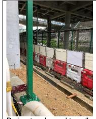
Perimeter channel to collect site runoff.
