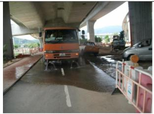
Silt was removed by water tanker.
