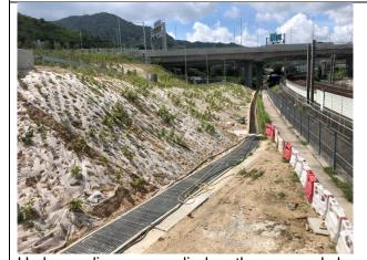
Hydroseeding was applied on the exposed slope.
