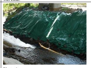
**Photo 6**Open slopes were covered with tarpaulin sheet as far as practicable to minimize muddy runoff.
