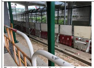
Perimeter channel to collect site runoff.
