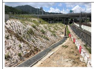
Hydroseeding was applied on the exposed slope.
