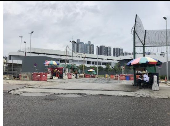
No wastewater flowing from the site to public area was observed.
