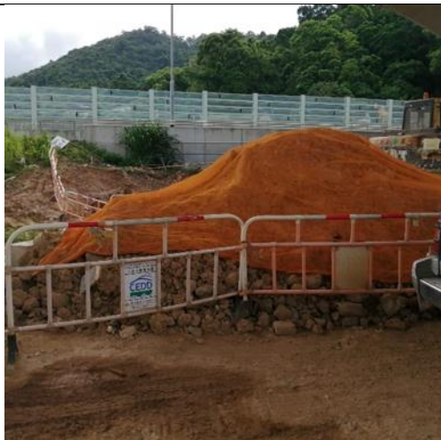
Stockpile was covered properly.
