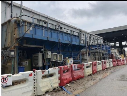
Wastewater treatment facility was implemented on site.
