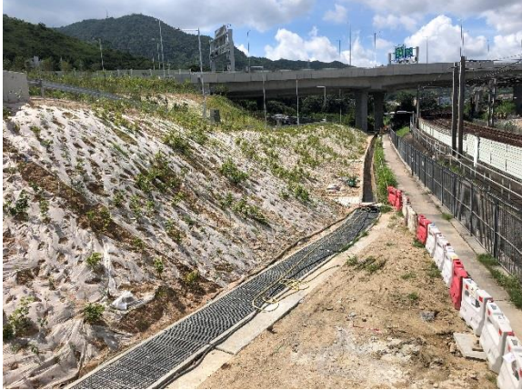
Hydroseeding was applied on the exposed slope.
