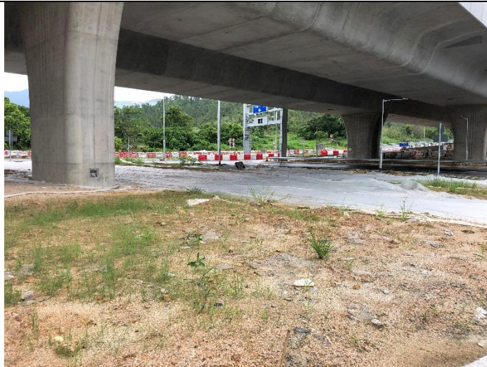
Hydroseeding was applied on the exposed surface.
